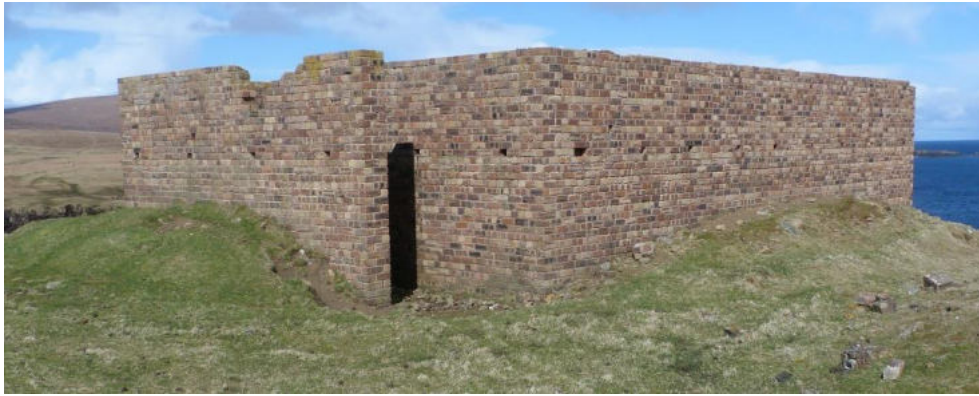
Plate 1: View of the external blast wall of the ACH Transmitter (Site 96) (From Carle, 2018a)
