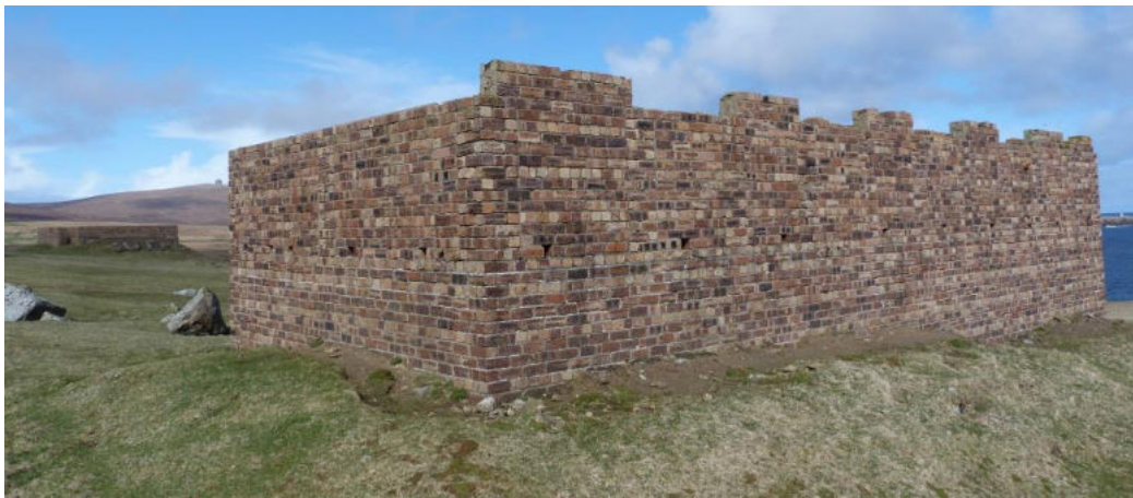
Plate 2: View of the external blast wall of the ACH Receiver (Site 99) (From Carle, 2018a)
