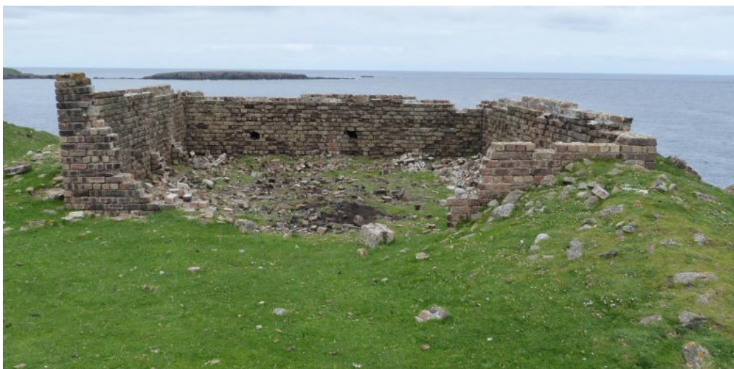
Plate 3: View of the external blast wall of the ACH Generator (Site 98) (From Carle, 2018a)
