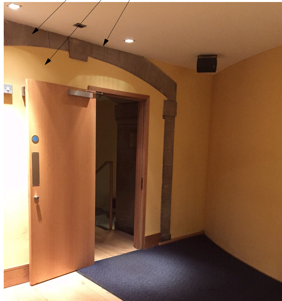
1 TO GF STORE WALL PHOTOGRAPH OF EXISTING MASONRY ARCH
