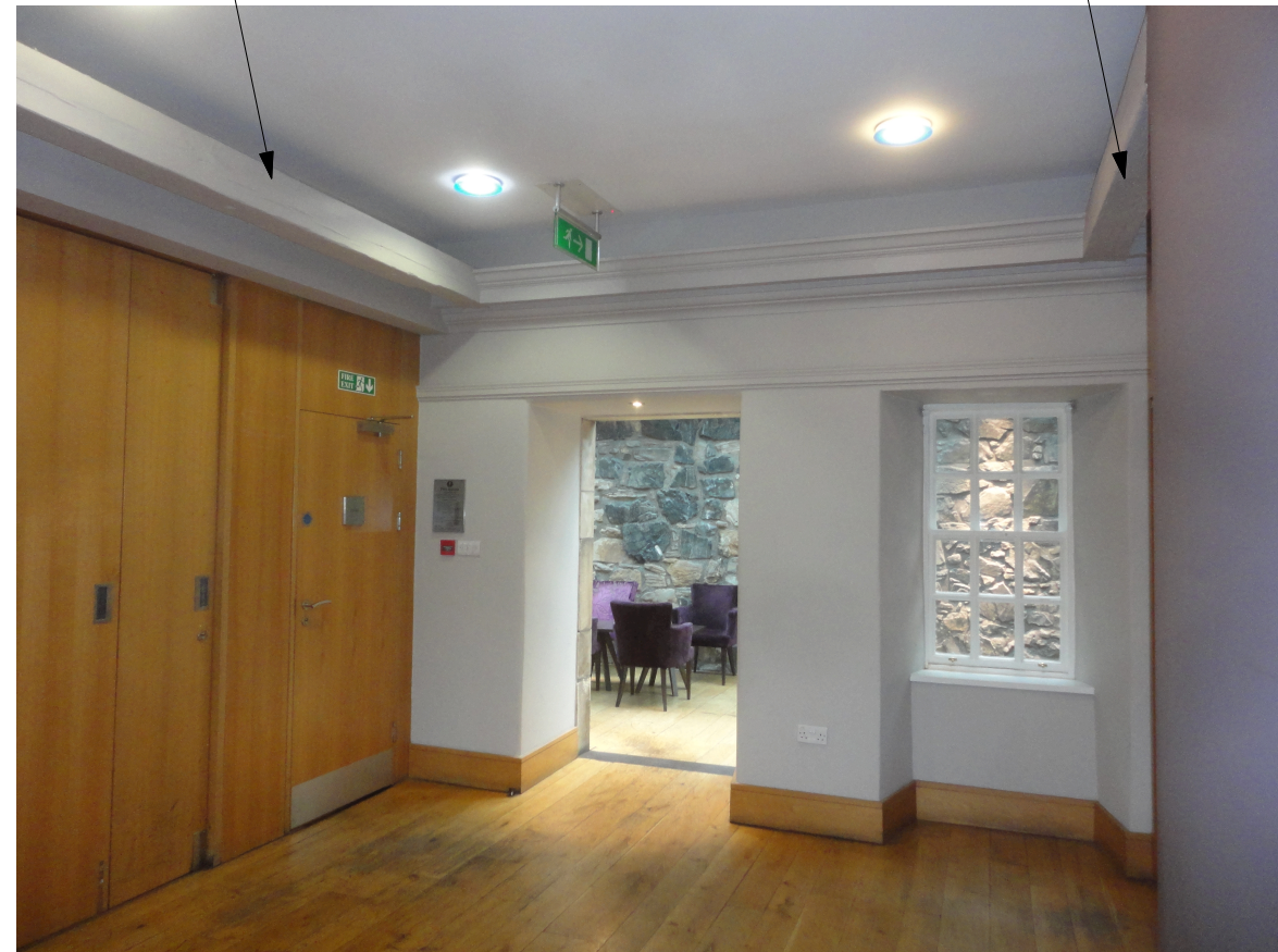
2 PHOTOGRAPH OF EXISTING BEAM AND COVING IN FF LOBBY NTS
