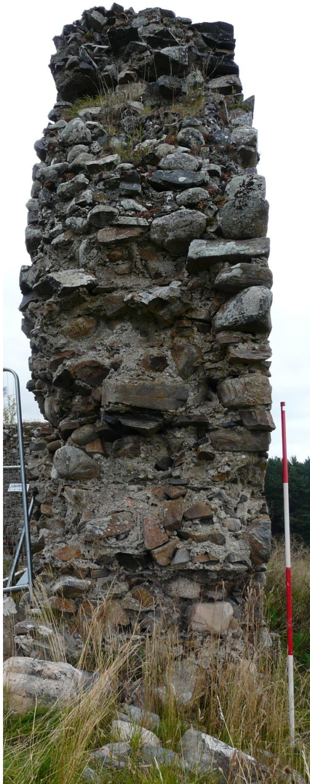
Figure 5 – Full face-core-face cross-section of south-east wall visible and accessible from breach in south corner. Note large volumes of core mortar. Scale 500mm; photograph M. Thacker.
