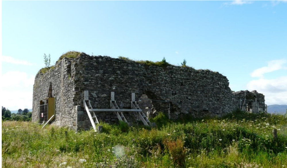
Figure 6 – Castle Roy from the north-north-west. Note north-east and north-west arch-headed entrances, exposed wall core at lower levels and around postern of the north-west wall, and some recent consolidation and temporary buttressing of northern tower. No Scale; photograph M. Thacker.
