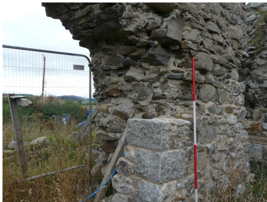
Figure 7 – Exposed primary core rubble of the north jamb of the north-west postern entrance, with some recent consolidation and re-facing of the internal face and jamb. Scale 500mm; photograph M. Thacker.
