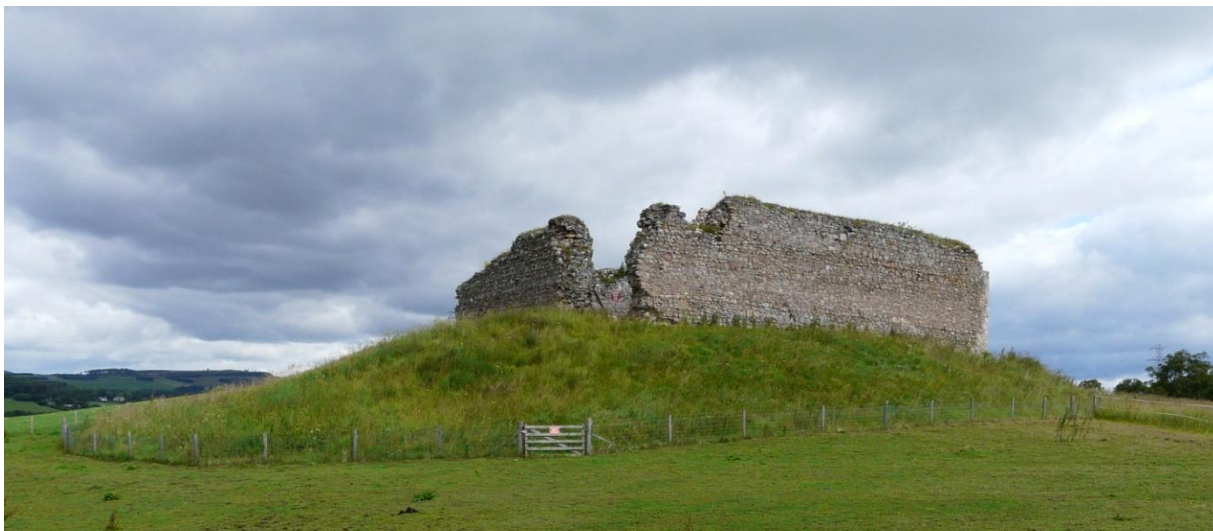
Figure 4 – From the south Castle Roy appears to be located atop a prominent mound. This view also shows the large breach and adjacent exposed wall cores at the south corner of the enclosure. No Scale; photograph M. Thacker.
