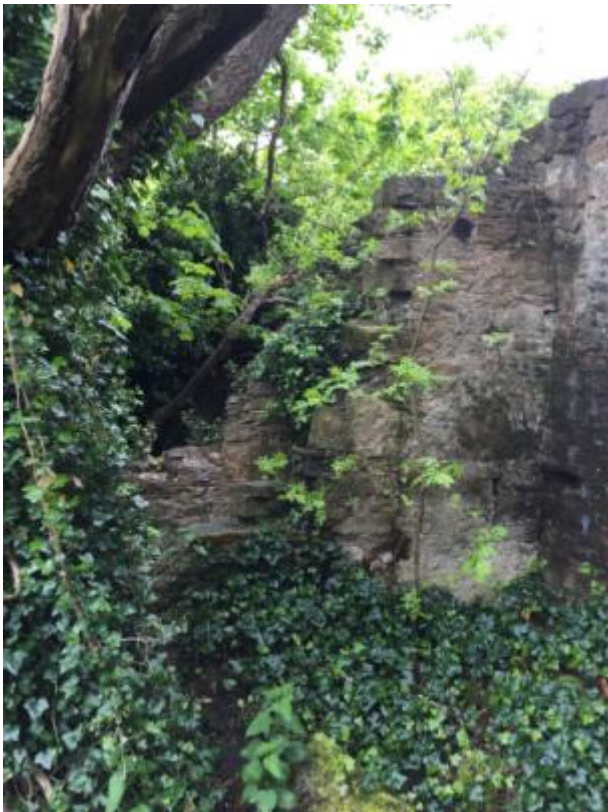
1: South Wall, South face
