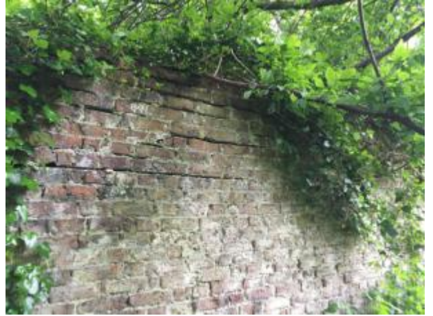
4: South Wall, North face Shows general condition of brickwork
