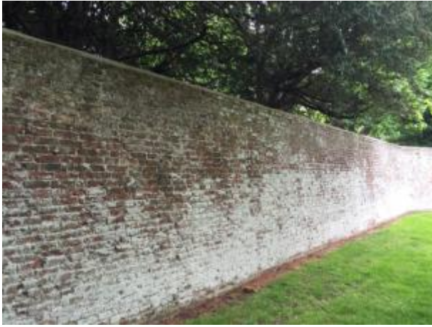
3: North/East corner, South face Lichen growth to brickwork surface
