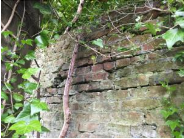
3: East wall, West face Vegetation growth, open mortar joints
