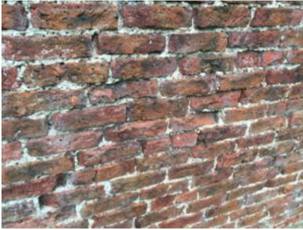
5: North Wall, South face Defective brickwork
