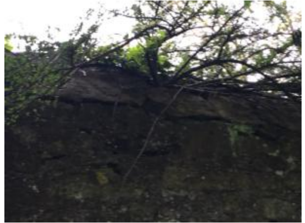
4: West Wall, East face
