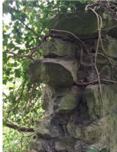
10: South Wall, South Face Close up of wall showing construction
