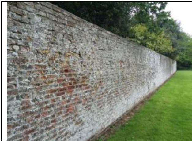
3: North/East corner, South face Lichen growth to brickwork surface
