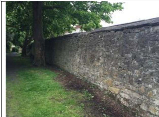
9: South Wall, South Face Excessive vegetation growth, partial collapse of wall
