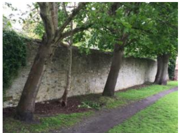
2: West Wall, East face General view of wall
