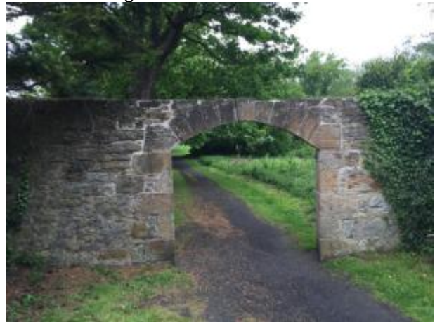
6: South Wall, South Face Shows opening at path
