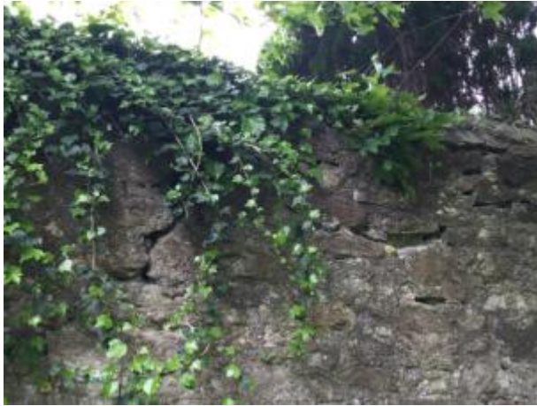
3: West Wall, East face
