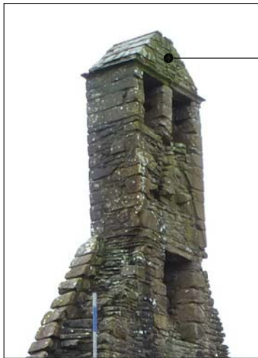
VIEW OF BELLCOTE AFTER REMOVAL OF CROSS & COPING SOCKET STONE.
