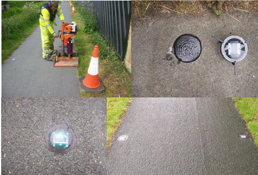
Fig. 2. Installation of LED's.
