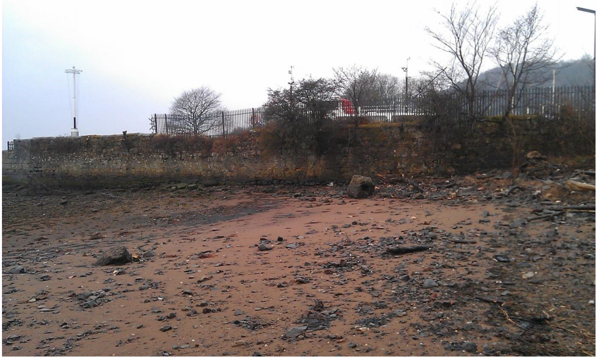
Retaining wall at low tide.
