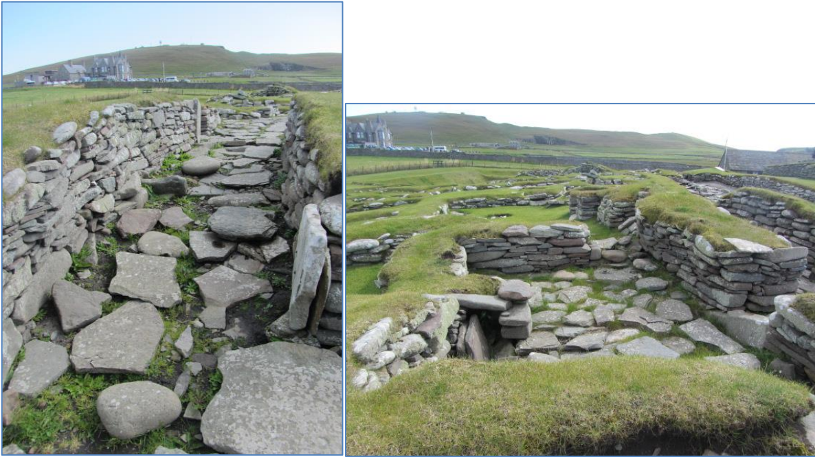
Figs 6 & 7. Examples of paved areas to be consolidated, vegetation removed and paving relayed and surrounded by fine gravel.
