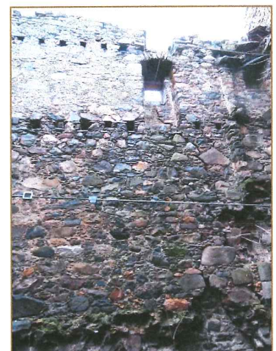
WEST WALL INTERNALLY - NOTE CORBELLING OVERHANG AND EXPOSED TO EROSION UPPER WINDOW ARCH; OTHERWISE, APART FROM USUAL EROSION THE WALL IS IN RELATIVELY GOOD CONDITION
