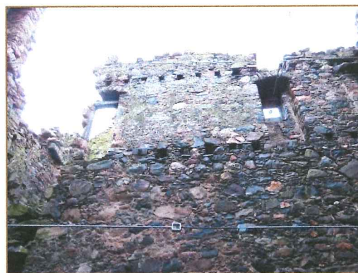
WEST WALL INTERNALLY - NOTE CORBELLING OVERHANG AND EXPOSED TO EROSION UPPER WINDOW ARCH; OTHERWISE, APART FROM USUAL EROSION THE WALL IS IN RELATIVELY GOOD CONDITION
