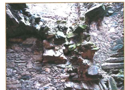
JUNCTION AT THE BEGINNING OF CIRCULAR STAIRS AT FIRST FLOOR
