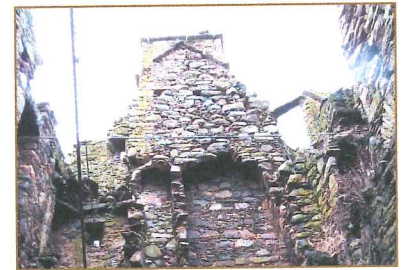
CHIMNEY SUPPORTED BY ARCHING MASONRY; THE ARCH SPANS BETWEEN TWO DELICATE AND HEAVILY ERODED PIERS
