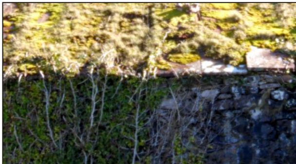
NORTH AISLE WEST WALLHEAD
