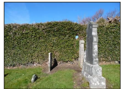
VIEW OF SOUTH WALL COVERED BY IVY
