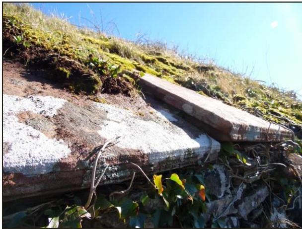
NORTH AISLE - ORIGINAL ROOFING SLABS LIFTED BY ROOTS, LOOSE WALLHEAD STONES HELD BY IVY
