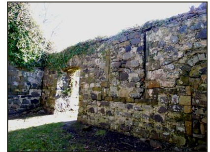
SOUTH WALL INTERNALLY – ABOVE AND BELOW - VISIBLE TILT AND DISTORTIONS AT INFILLS
