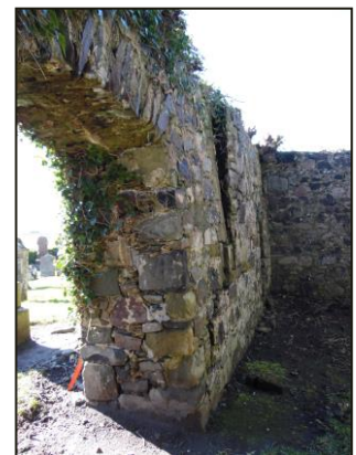
SOUTH WALL INTERNALLY – ABOVE AND BELOW - VISIBLE TILT AND DISTORTIONS AT INFILLS
