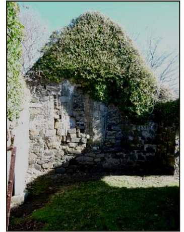
EAST WALL WITH ELABORATE WINDOW OBSCURED BY IVY
