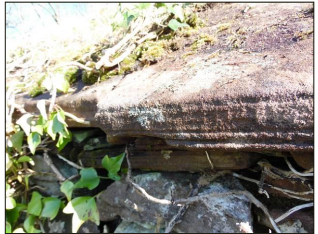
NORTH AISLE - ORIGINAL ROOFING SLABS LIFTED BY ROOTS, LOOSE WALLHEAD STONES HELD BY IVY
