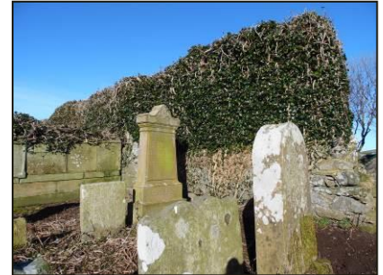
SOUTH WALL OVERGROWN WITH IVY
