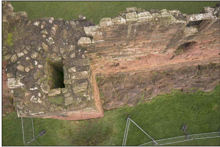
ROUGH RACKED WALLHEAD TO LATRINE TOWER: photographed 13th March 2015
