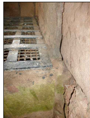
Defective and corroded yett fixings. Fixings to be cut out to allow removal of yett, with new fixings into stonework joints being used to re-install yett once condition inspection of shaft and any necessary repairs have been completed.
