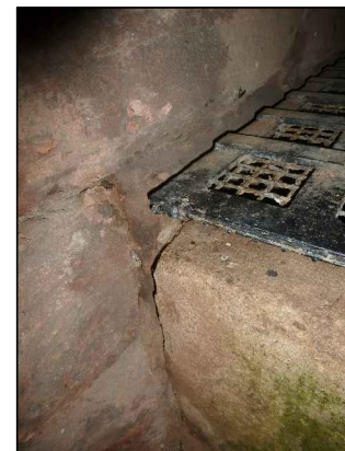
Defective and corroded yett fixings. Fixings to be cut out to allow removal of yett, with new fixings into stonework joints being used to re-install yett once condition inspection of shaft and any necessary repairs have been completed.
