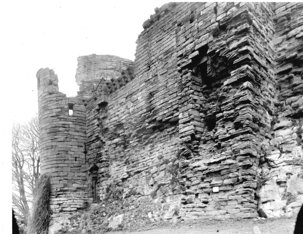
1 Photo believed to date from c.1899 showing Latrine tower prior to early C20 consolidation work
