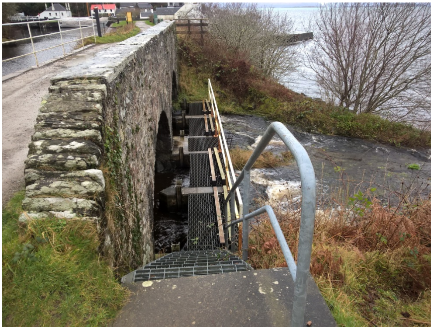
Crinan Weir – Ducting to cross on steel walkway and not over historic masonry structure.
