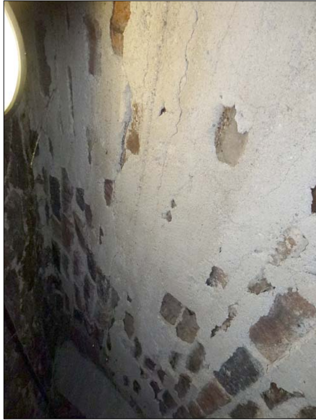
Continuous cracks to mortar bed joint and bulge to brickwork.
