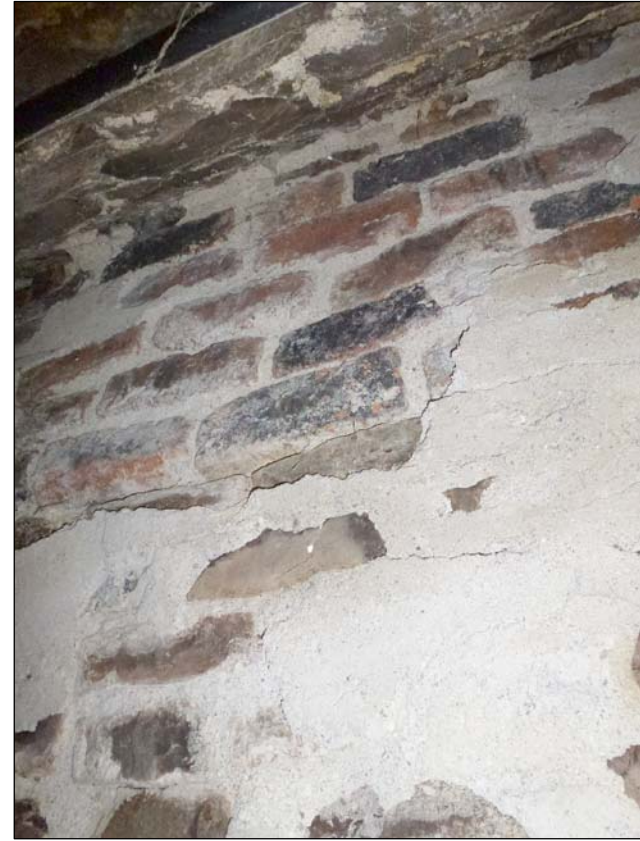
Hungry joints to brickwork and areas of adhered mortar from bricks being built off shuttering.
