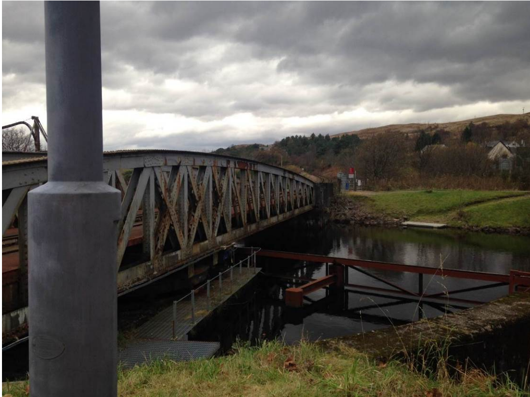
Photograph 1: bridge in closed position – showing existing walkway
