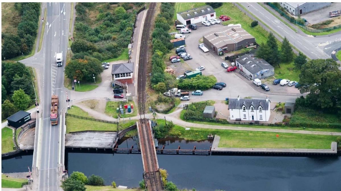
Photograph 6: Railway Swing Bridge – looking to the SE
