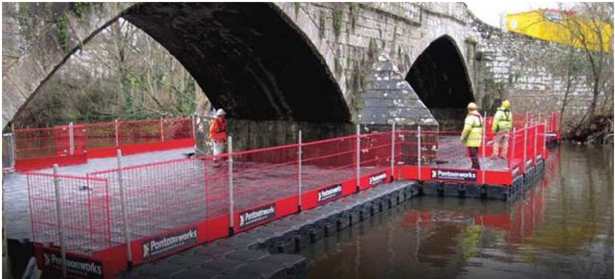
Photograph 5: example of pontoon in use
