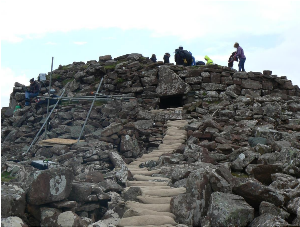
Figure 1: Conservation works at the broch in 2012.
