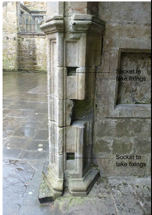
Photo 2 showing open sockets to take new gates.
