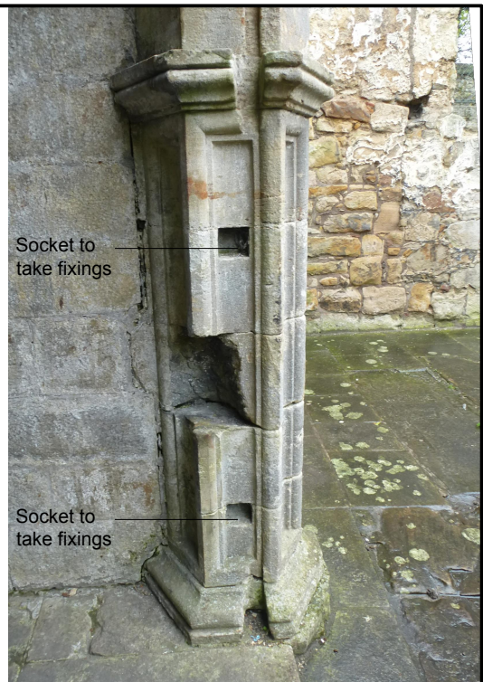
Photo 1 showing open sockets to take new gates.
