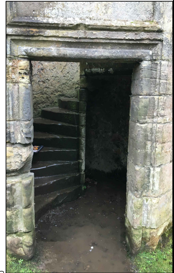
Photo showing opening up to Lairds Loft
