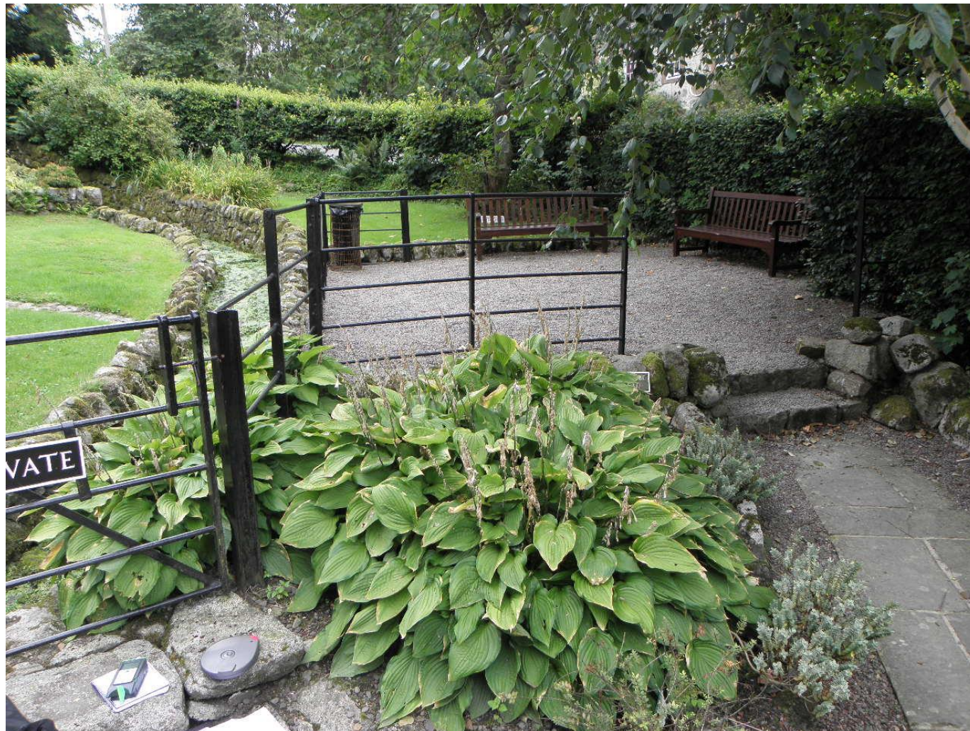
1. General view of garden area adjacent to west of Mill building before hedge was breached. The rubble wall and steps creating the gravelled viewing area terrace and estate railings are all 1980s or later in date.
