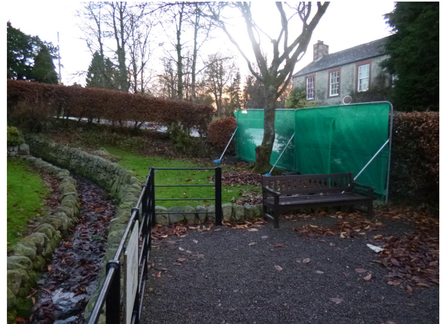
11. View of garden area adjacent to west of Mill building showing breached hedge, damaged cherry tree and area where ground would be reprofiled under submitted proposals.
