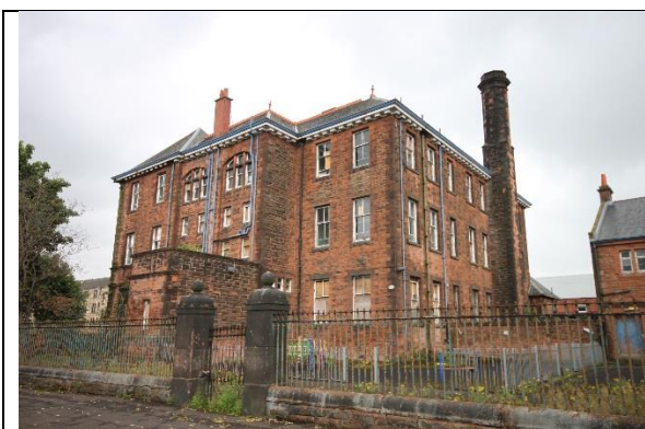
Greenfield Primary School and Swimming Baths, west elevation, looking northeast. (03/08/2016) © Historic Environment Scotland
