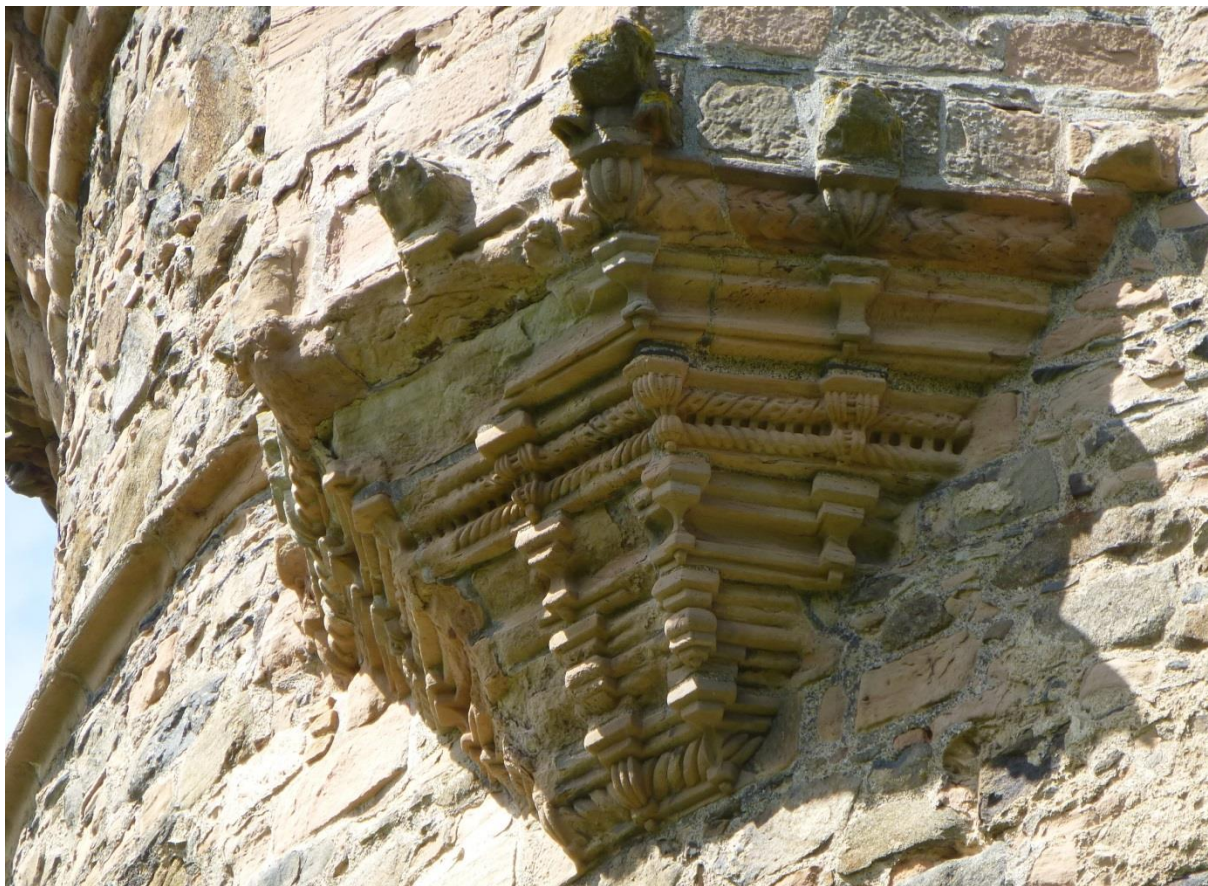
Oriel Window of South tower – east face
