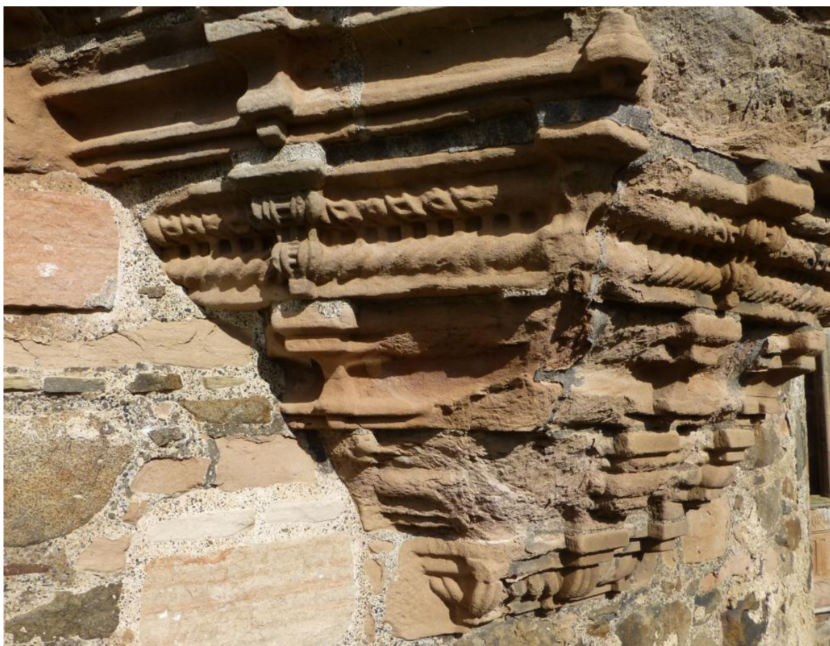
Oriel Window of South tower – west face
