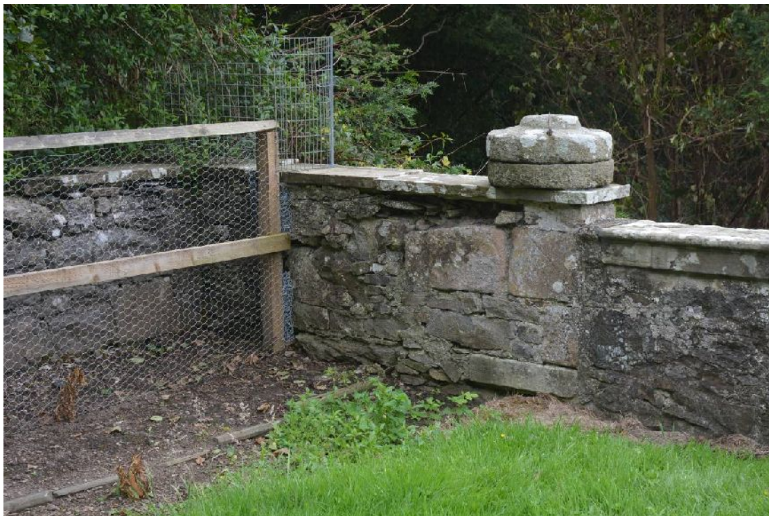
Illus 37 SE corner of Terrace showing difference in structure between E wall and the upper part of the N garden wall bordering the S side of the Terrace. Note the raised part of this wall is over the differently constructed retaining wall of the lower House Terrace
