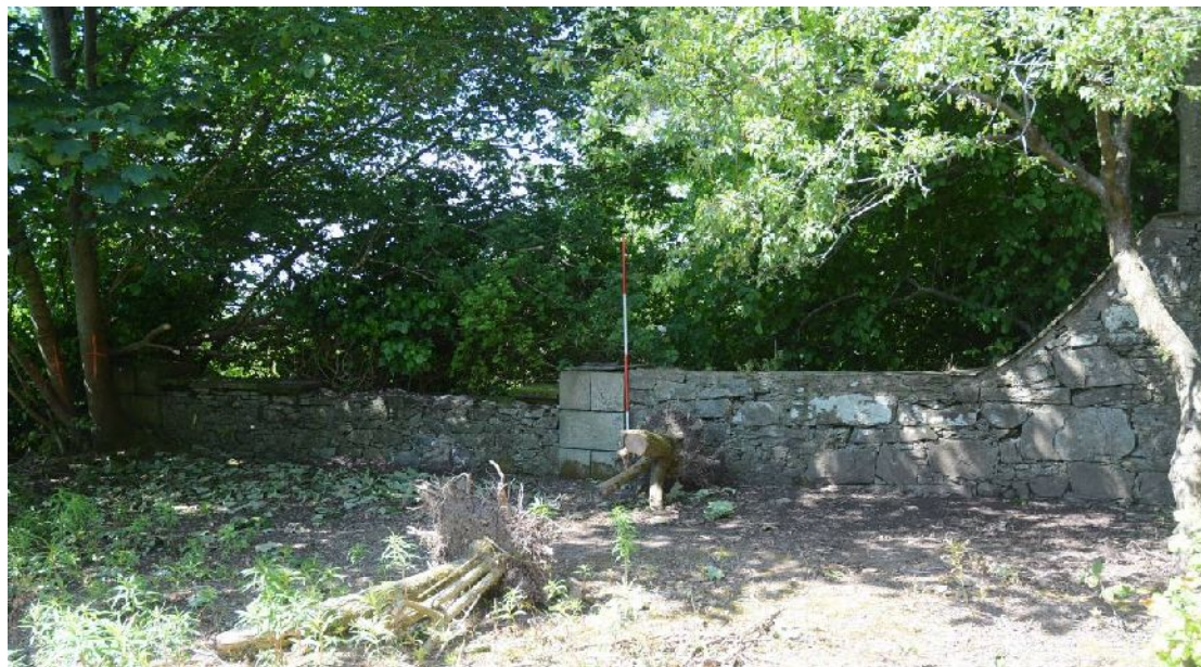
Illus 35 W wall of Terrace
