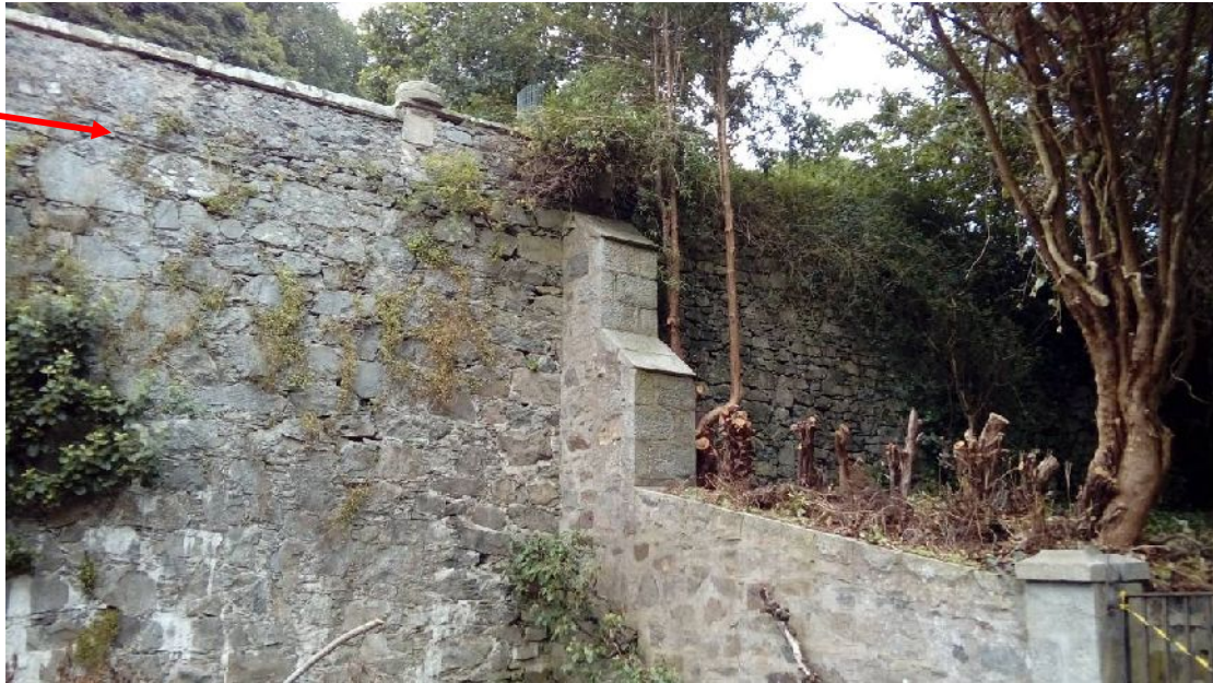
Illus 17 NE corner of walled garden at junction with E wall and showing differences in wall structure (red arrow). Note also the different structure to the E on the retaining wall of the House Terrace.
