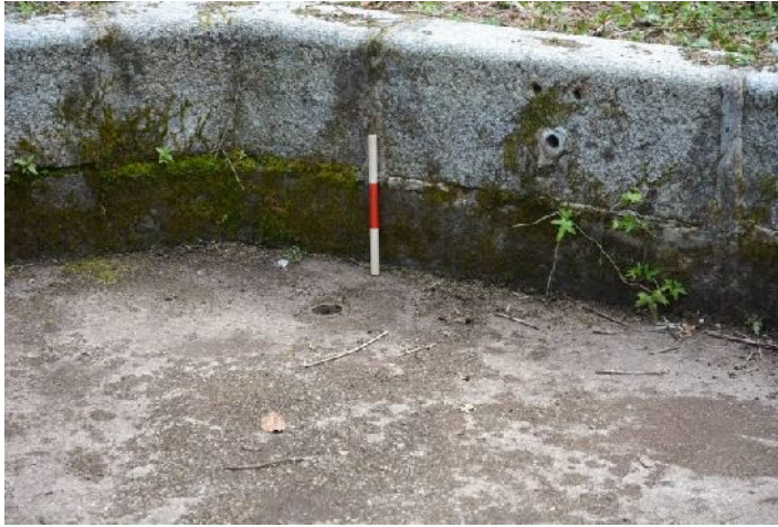
Illus 120 Fountain (8). Detail of outflow and drain.
