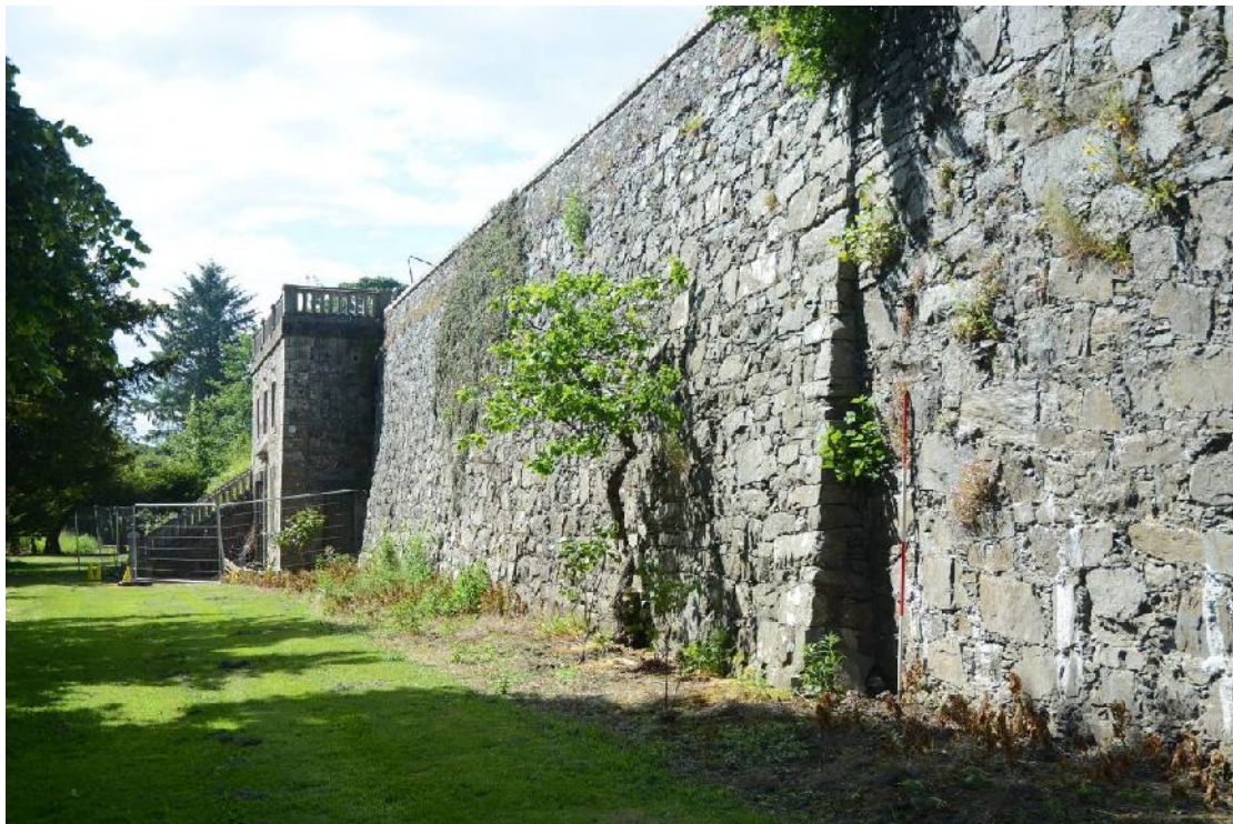
Illus 18 N wall E of Garden House, looking W, detail of buttress
