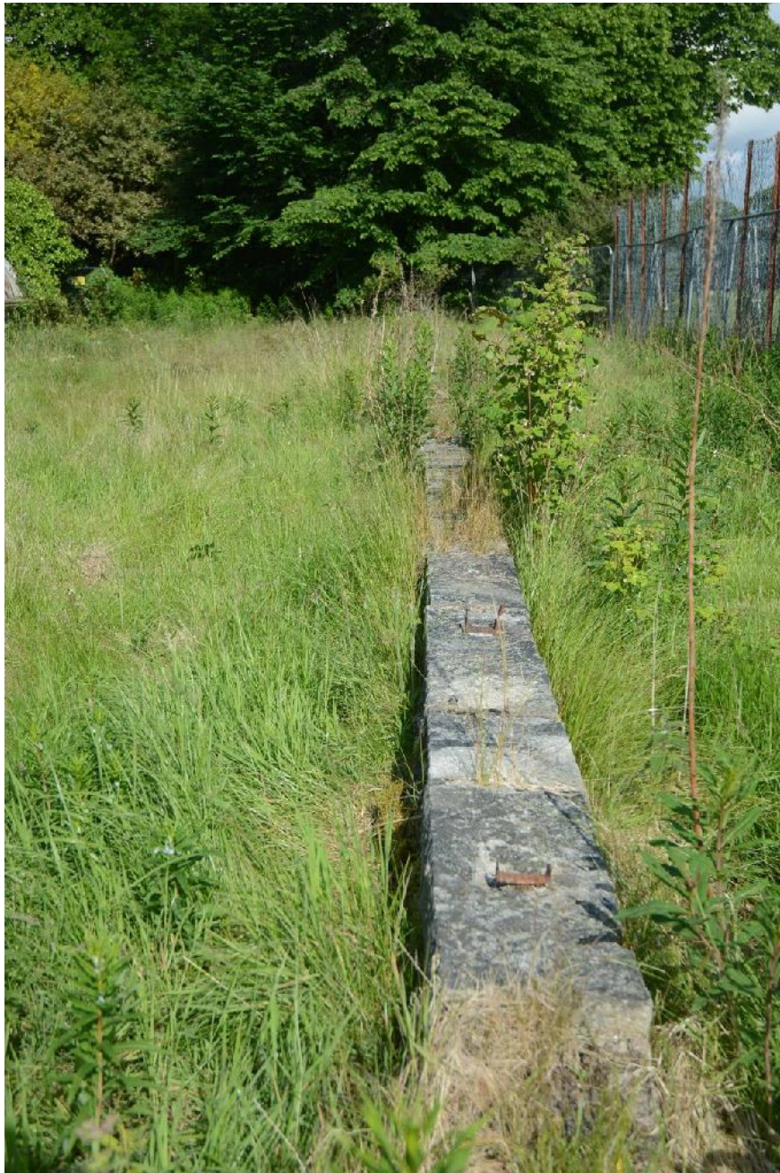
Illus 100 wall 29 looking E
