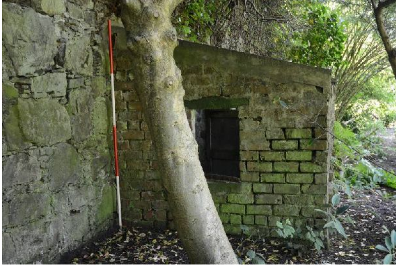
Illus 102 Building 17, E end
