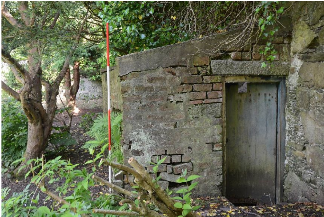
Illus 101 Building 17, W end
