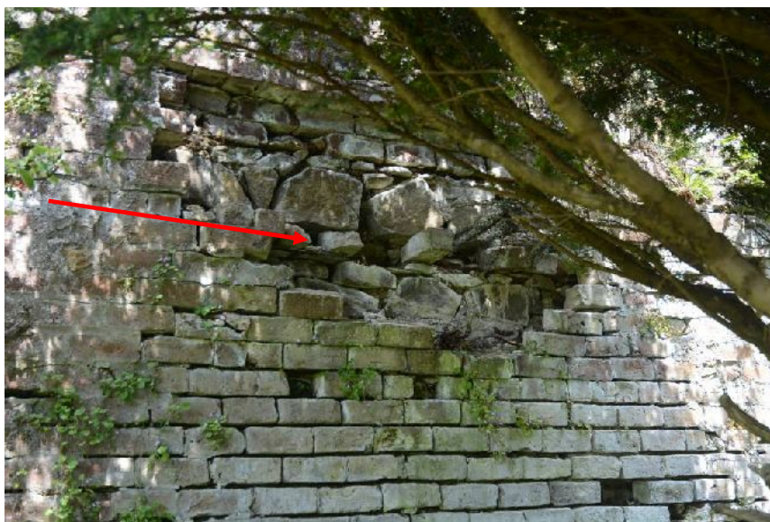
Illus 14 Detail of N wall W of Garden House. Red arrow marks line of tie-in bricks between inner brick facing and outer stone wall.
