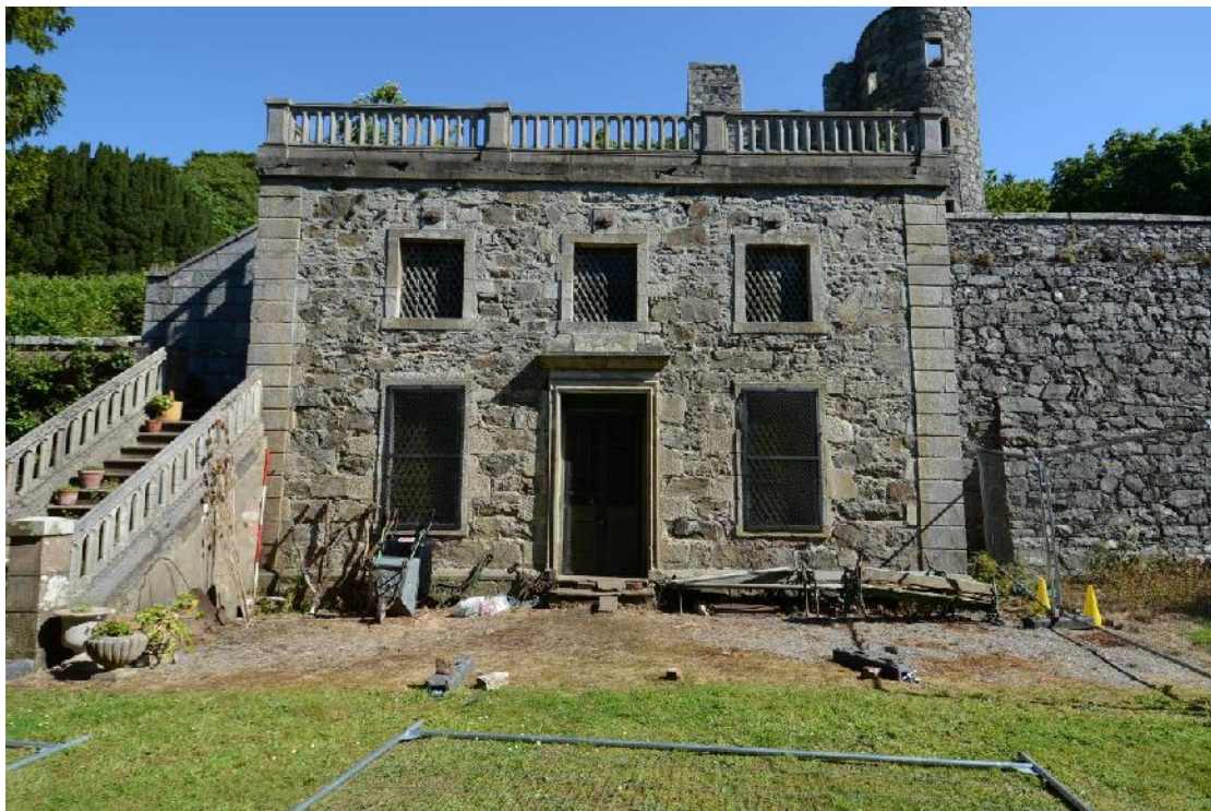
Illus 56 S facade of garden house.
