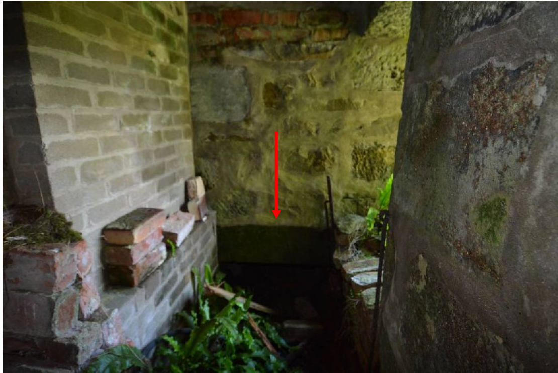
Illus 73 Arrow shows channel below steps
