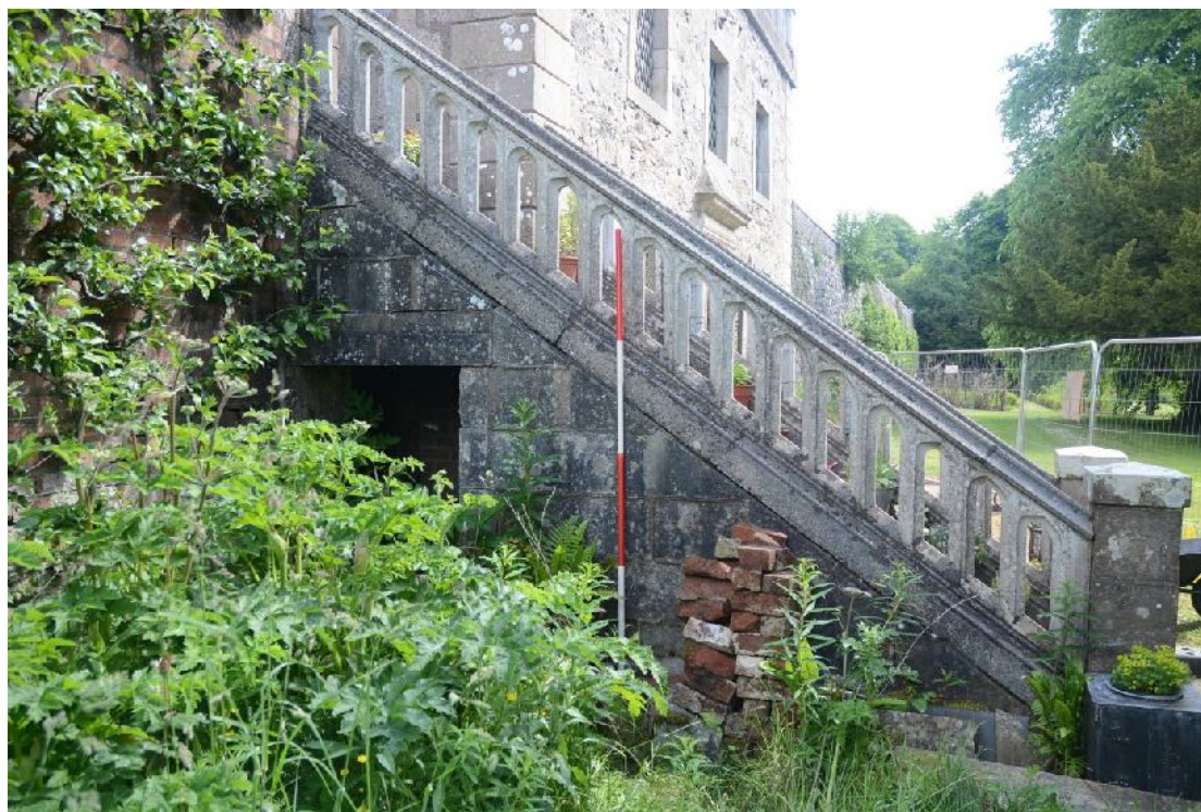
Illus 71 W side of steps showing doorway giving access to under-stair chamber
