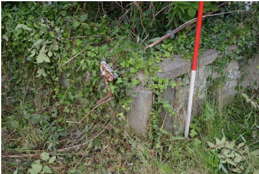
Illus 80 Greenhouse (27) SW corner showing stonework and winding mechanism
