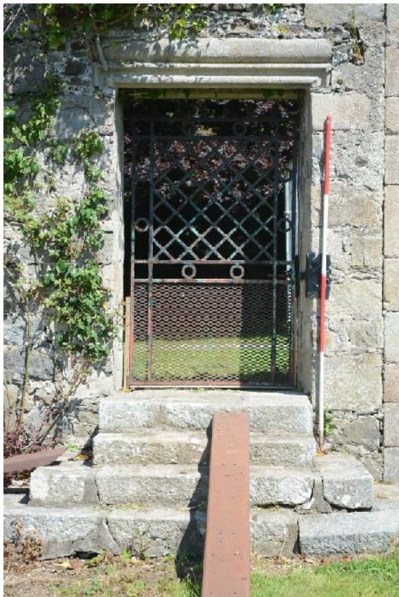
Illus 42 Garden door 3 internally, with re-used stone as lintel
