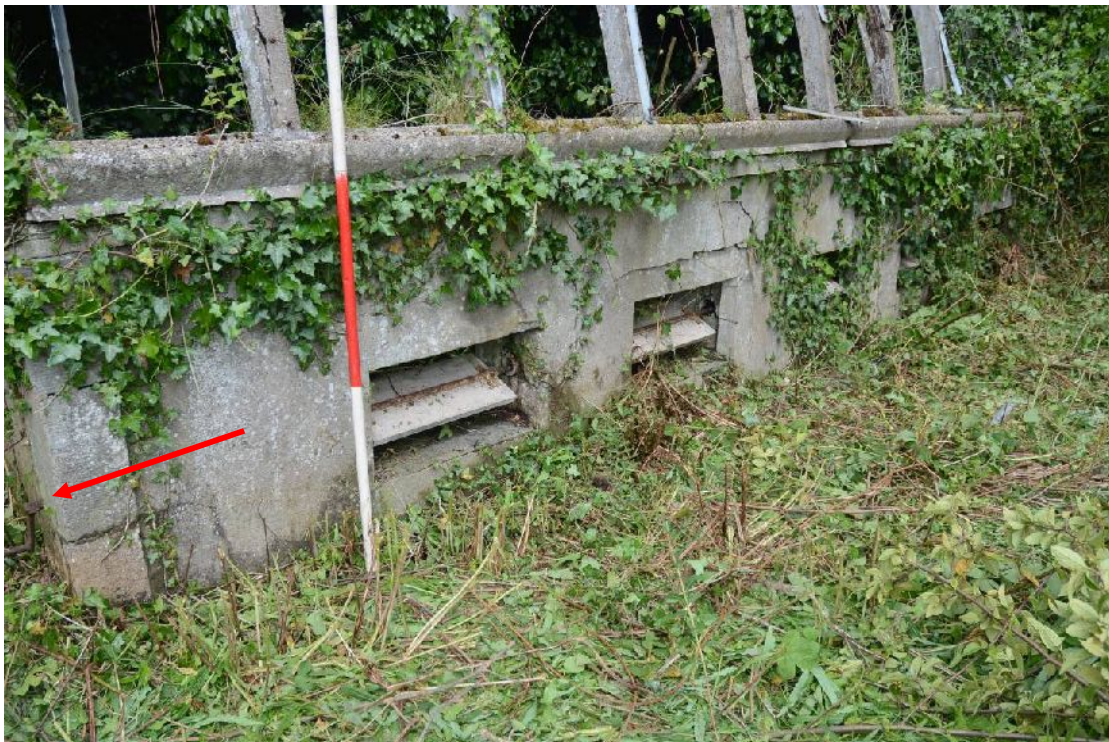
Illus 94 Original wooden vents. Winding handle visible on LHS
