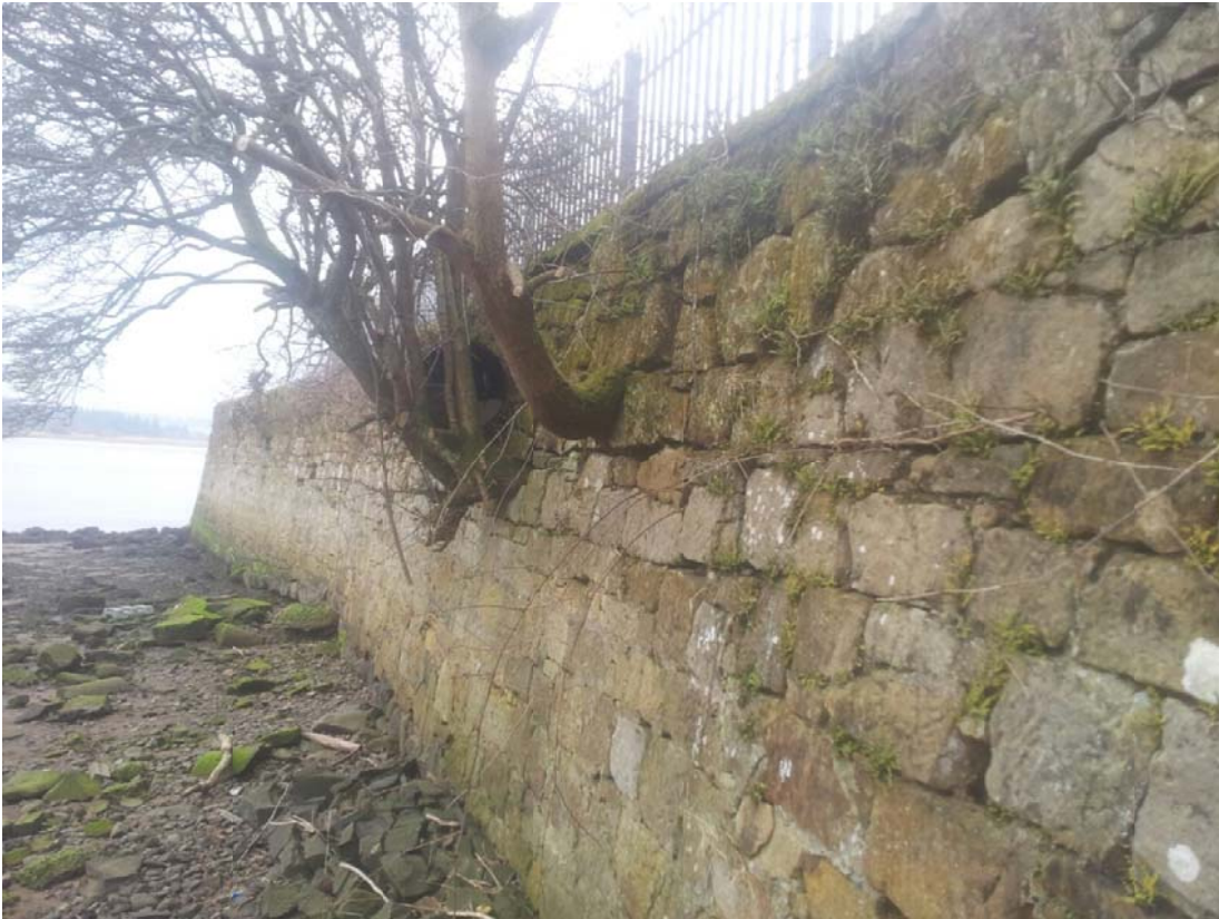
Picture 4 – Extent of rip rap to prevent undercutting
