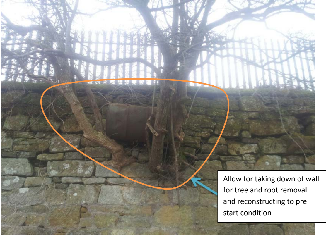
Picture 3 - Tree removal and wall reconstruction
