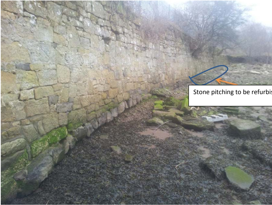
Picture 5 – Extent of existing stone pitching
