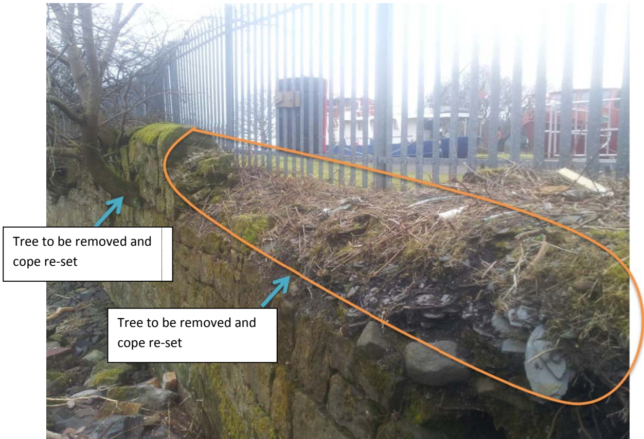
Picture 7 – Parapet reinstatement and tree removal
