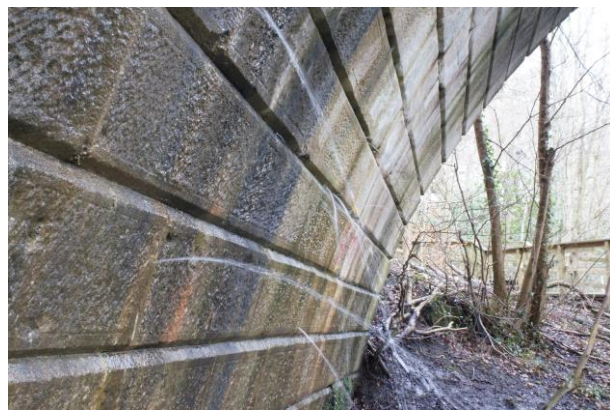
Avon aqueduct showing leakage exiting structure under pressure
