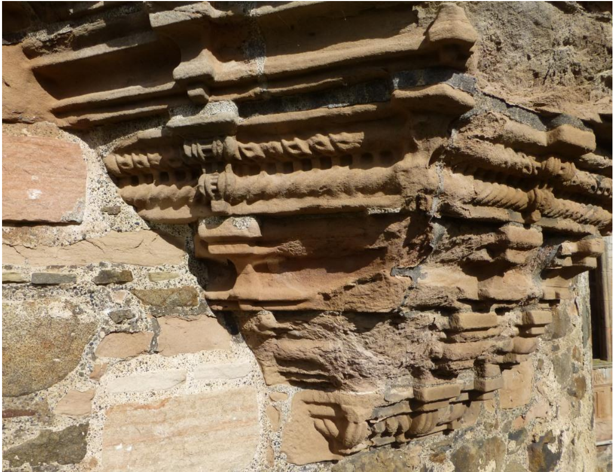
Oriel Window of South tower – west face
