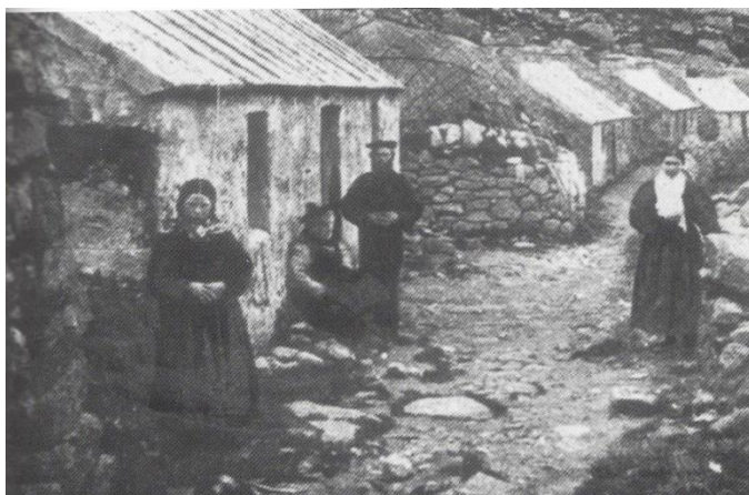
Figure 5 House 8 with blackhouses H and G behind 1883 (D Whyte in Emery p103)
