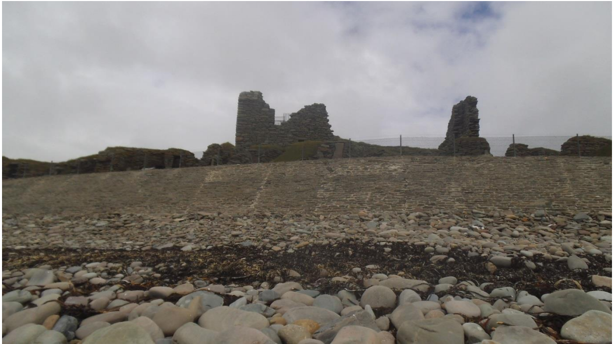
3. Regular lines where pointing is failing at wall panel joints
