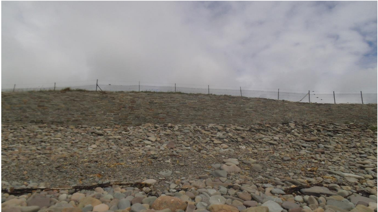
5. Less work appear required towards the west end of the wall (but see below)
