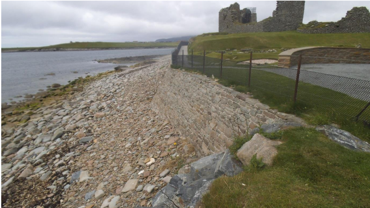
1. Start of sea wall adjacent to Visitor Centre
