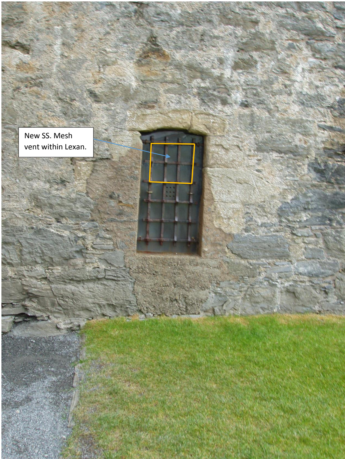
Typical yett installation with polycarbonate sheet (Lexan) behind to stop wind scour, litter and cat ingress.
