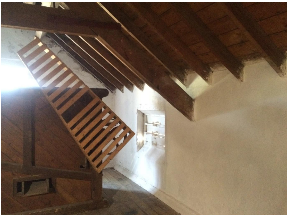
Area of inspection
