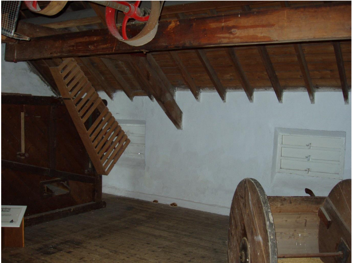
Barley Loft above malting floor. Plaster to be removed to allow access to rafters for treatment or renewal (in line splice). Louvred vent frames can hopefully be treated and retained. MCU to re-plaster and limewash on completion.
