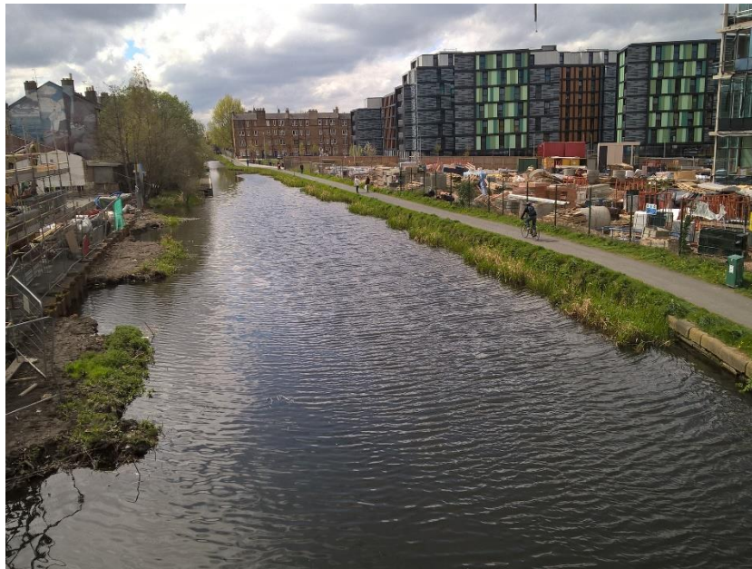
Fig 2. The strip vegetation strip will be removed and the towpath setts extended to the canal wall.
