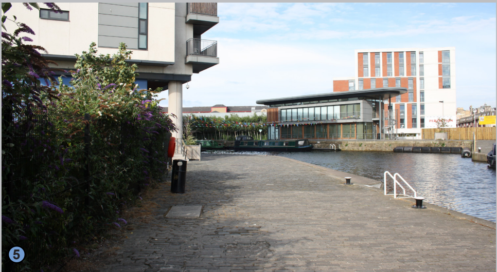
View 5, Looking North East along Union Canal, showing existing canal quayside.
