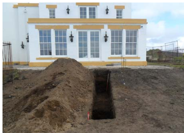
Plate 2: Re-excavated 2008 evaluation trench
