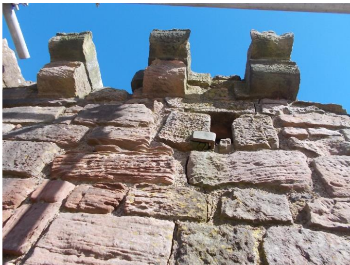
Architectural details at the wallhead. An opportunity can be taken to examine these during the works.
