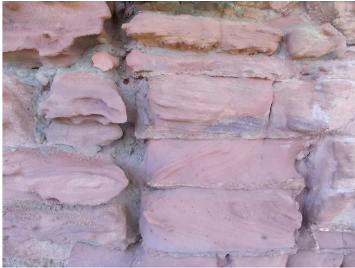
Detail of eroded stonework, probably representing early 20 th -century repairs
