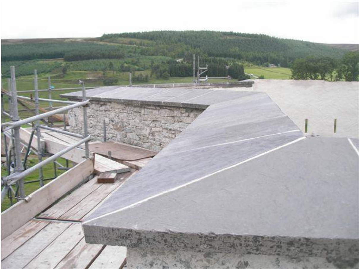
New copes being placed to south wall 2010
