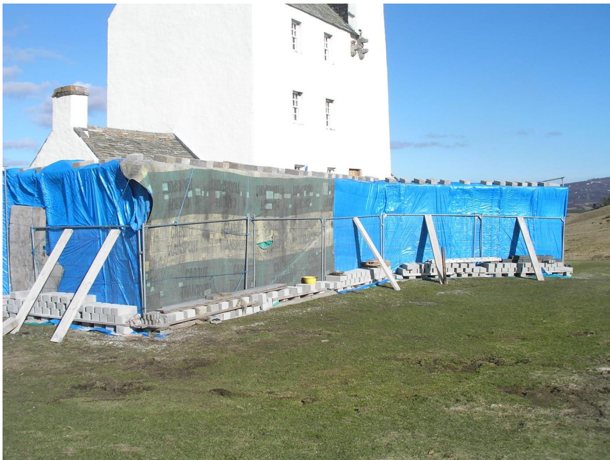
Renewal of lime harl to south outer wall in progress 2010
