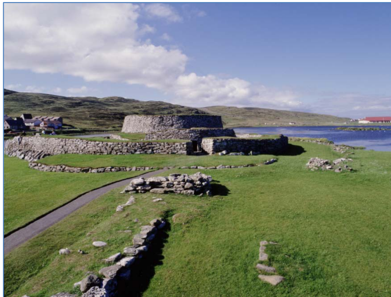
Fig 3. Clickimin today, following excavation, reconstruction and consolidation.
