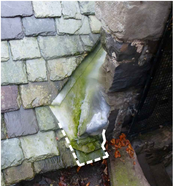
Photo 3 - Extend Lead Flashing, tuck under existing flashing.
