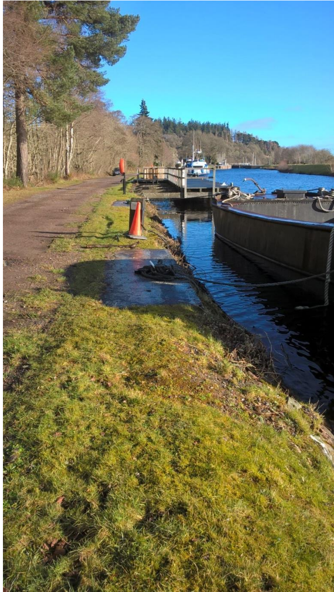
Fig 3. Showing Concrete Blocks to be removed.
