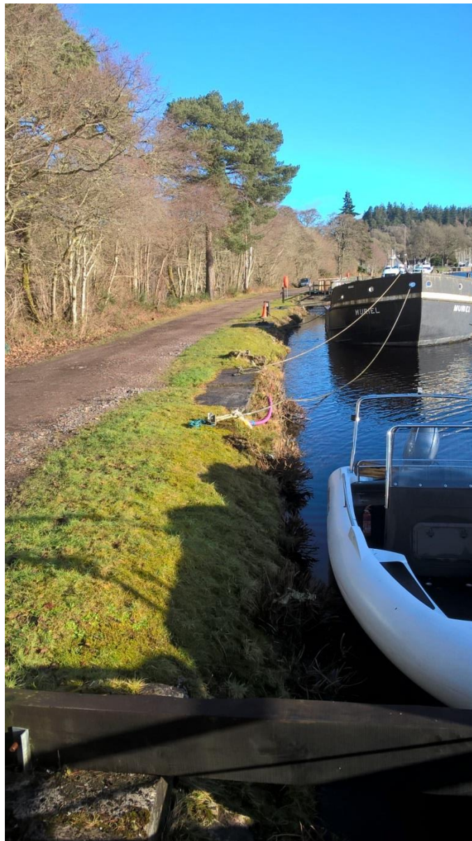
Fig. 2. Showing Concrete Block to be removed.
