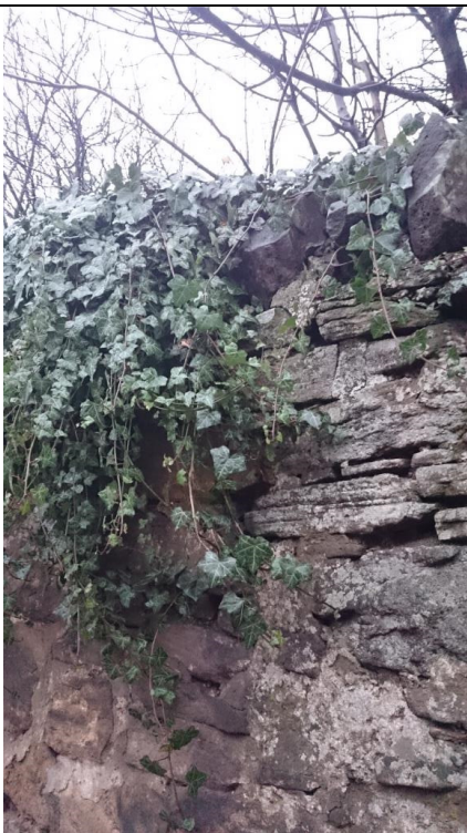
Photo 07: Boundary wall on Old Dalkeith Road
