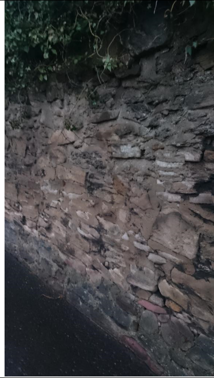
Photo 10: Boundary wall on Old Dalkeith Road
