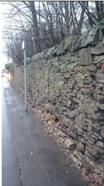
Photo 06: Boundary wall on Old Dalkeith Road
