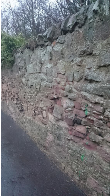
Photo 09: Boundary wall on Old Dalkeith Road
