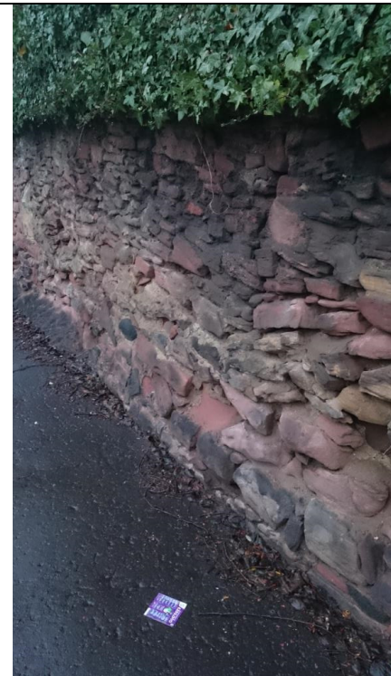
Photo 16: Boundary wall on Old Dalkeith Road
