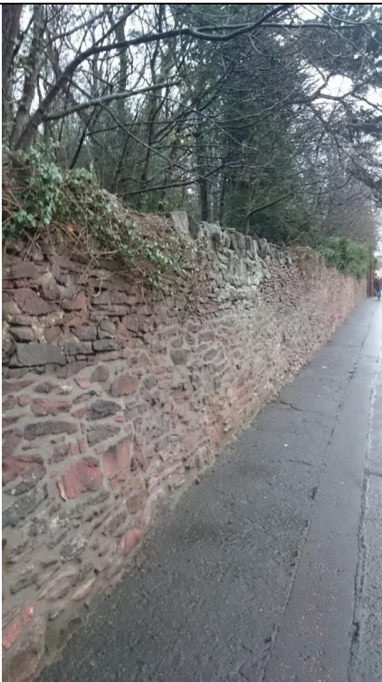
Photo 05: Boundary wall on Old Dalkeith Road
