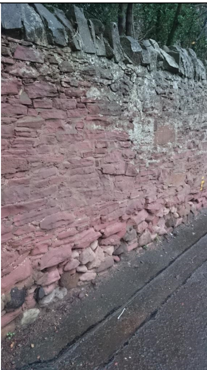
Photo 01: Boundary wall on Old Dalkeith Road
