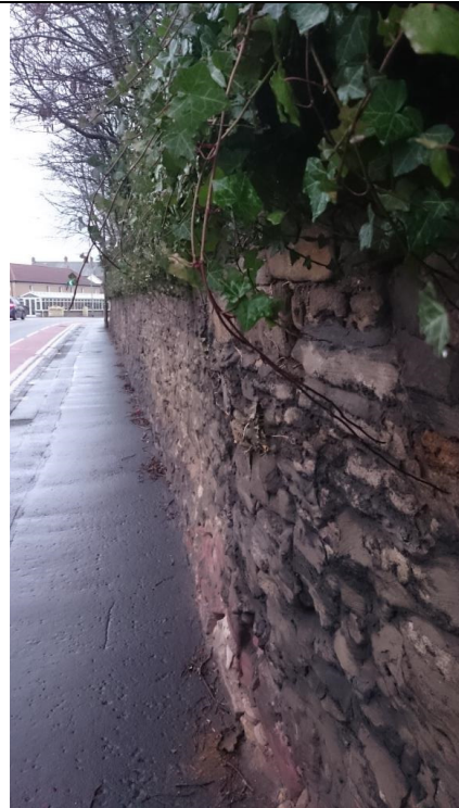
Photo 12: Boundary wall on Old Dalkeith Road
