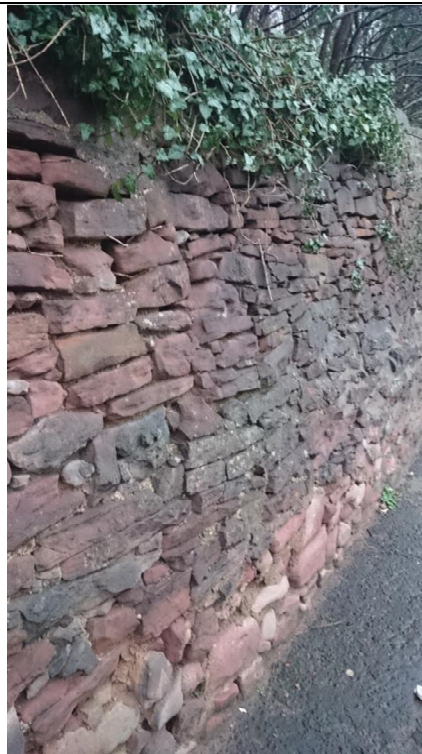
Photo 04: Boundary wall on Old Dalkeith Road
