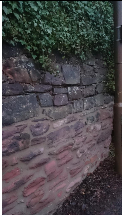
Photo 18: Boundary wall on Old Dalkeith Road
