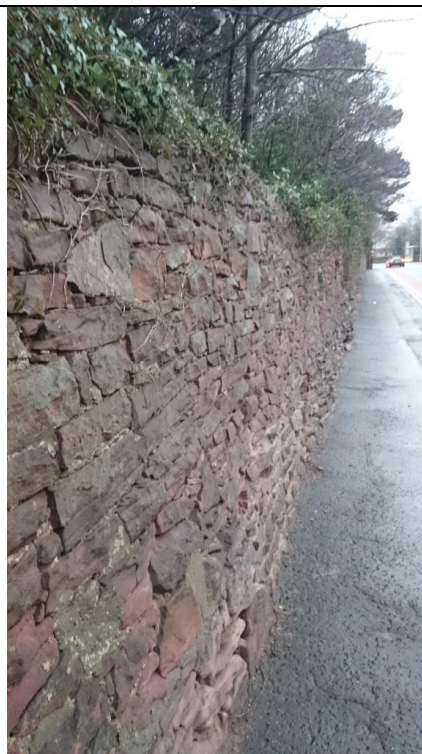
Photo 02: Boundary wall on Old Dalkeith Road
