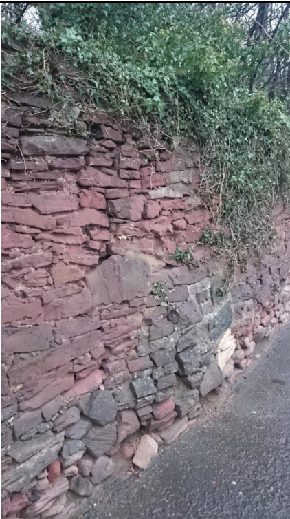
Photo 03: Boundary wall on Old Dalkeith Road
