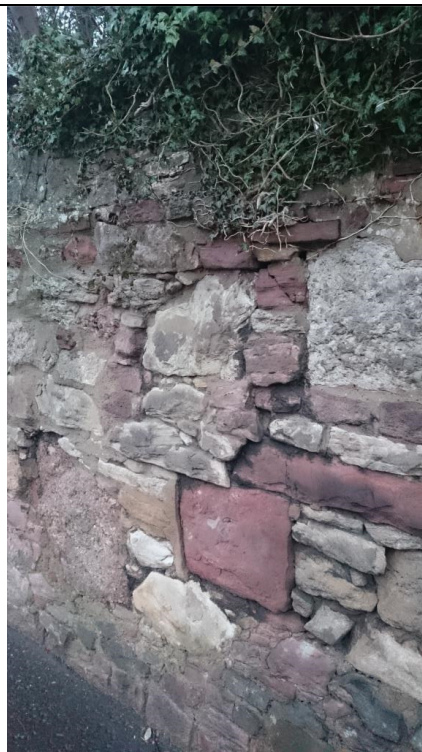
Photo 08: Boundary wall on Old Dalkeith Road
