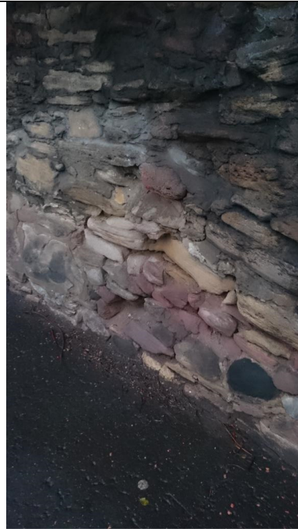
Photo 14: Boundary wall on Old Dalkeith Road
