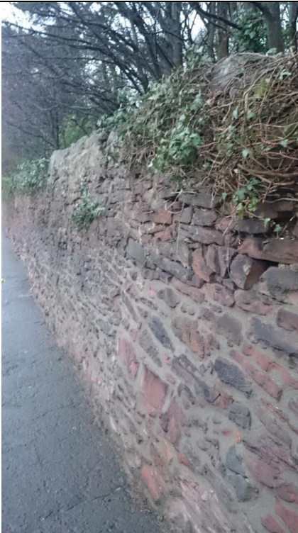
Photo 21: Boundary wall on Old Dalkeith Road
