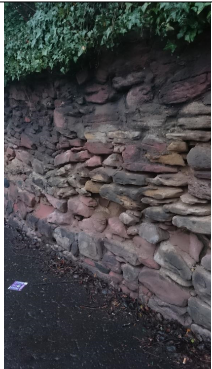
Photo 15: Boundary wall on Old Dalkeith Road
