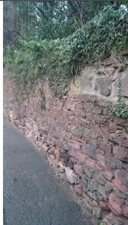
Photo 22: Boundary wall on Old Dalkeith Road
