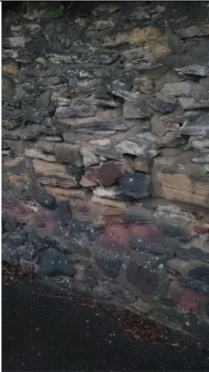
Photo 13: Boundary wall on Old Dalkeith Road
