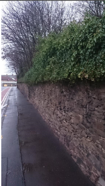
Photo 11: Boundary wall on Old Dalkeith Road
