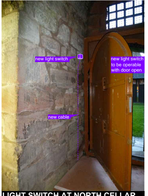
LIGHT SWITCH AT NORTH CELLAR diagrammatic view at door opening (Middle Cellar similar)
