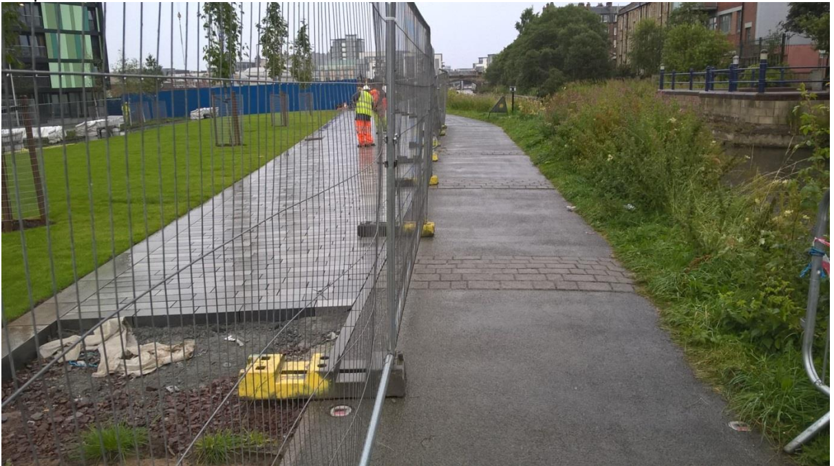
Photograph 1. Existing towpath and granite setts within the boundary of Boroughmuir High School. The towpath will be re-laid as setts similar to those within the school grounds. The towpath will be finished with edging stones and LED lights, which will keep the towpath visually distinct.
