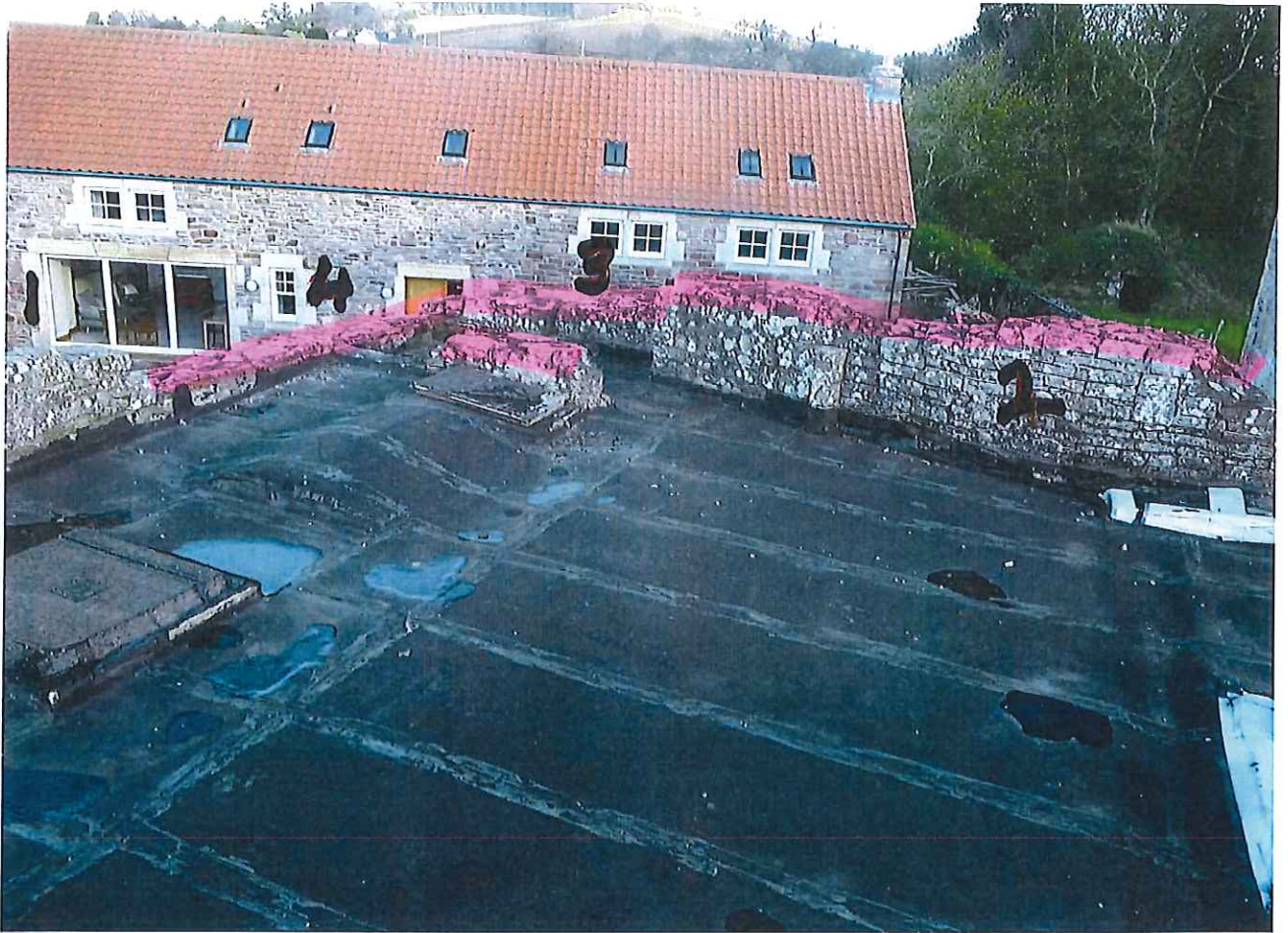
BALMERINO ABBEY, PARLOR RANGE FIRST FLOOR LOOKING EAST.
