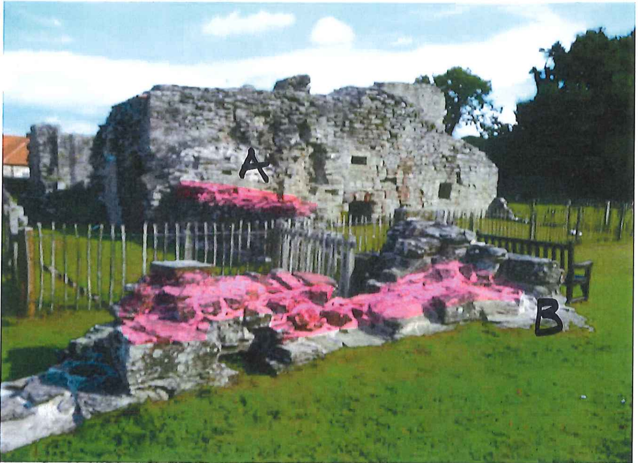
BALMERINO ABBEY. SOFT CAPPING TRIAL. LOW LEVEL TRIAL AREAS.
