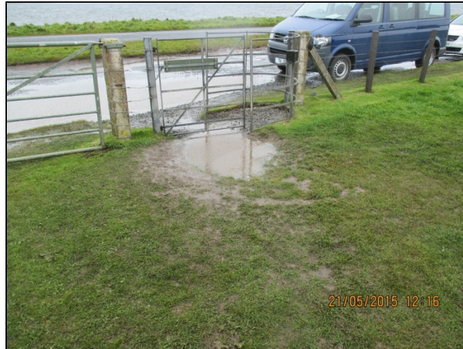
Plate 2: Car park access gate.
