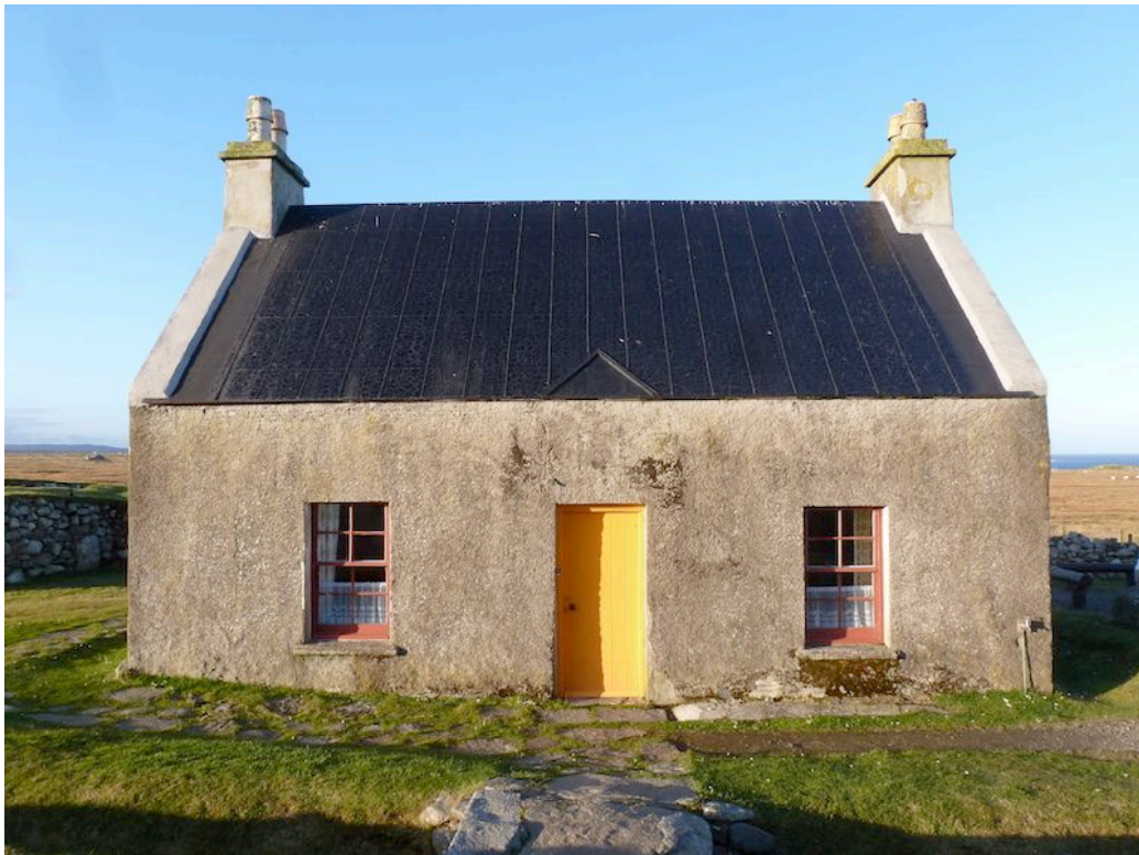
Photograph 4: East side of White house
