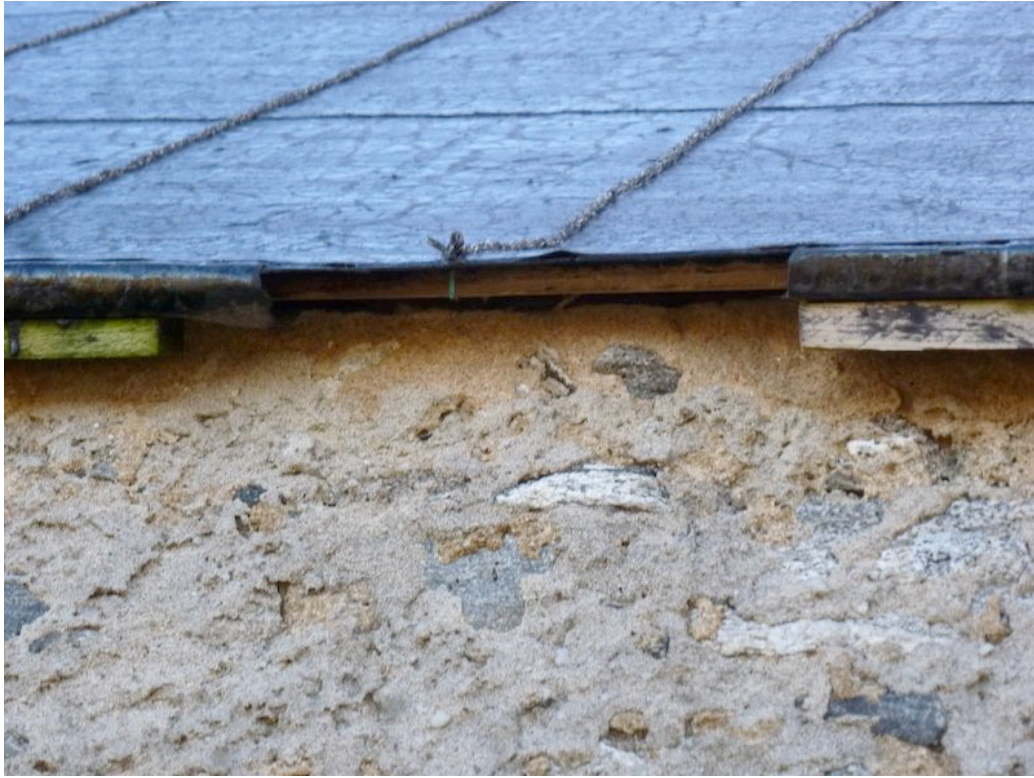
Photograph 5: West facing roof and wall of the white house
