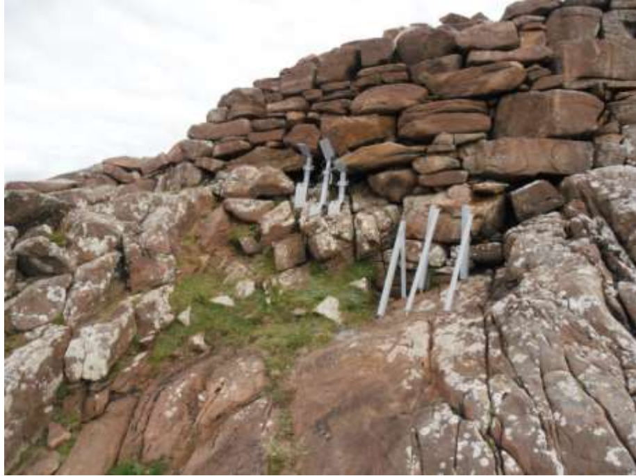
Figure 4: Temporary consolidation works to the South
