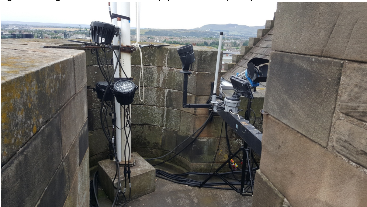
Fig. 4a Edinburgh Castle Gatehouse roof equipment location (South)
