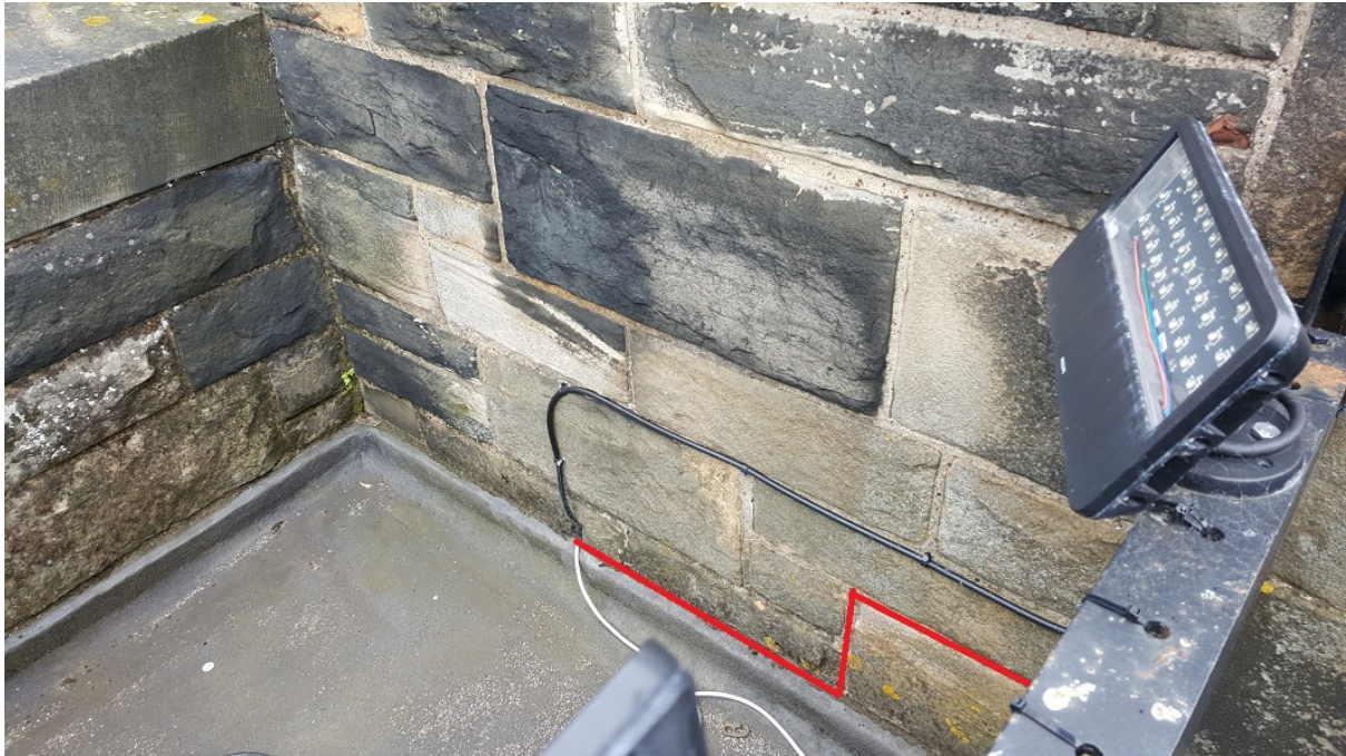
Fig. 6 Edinburgh Castle Gatehouse proposed cable run (South)
