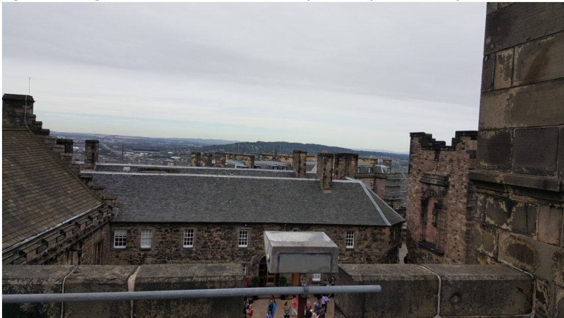
Fig. 22 Edinburgh Castle Palace roof west: access point and point to multipoint location
