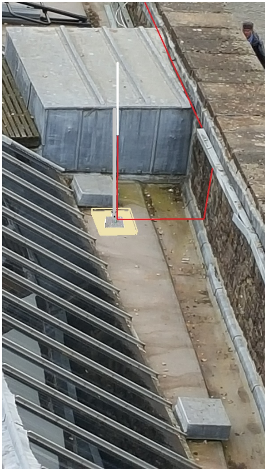
Fig. 11 Edinburgh Castle Gift Shop roof showing proposed antenna access point mount and cable run
