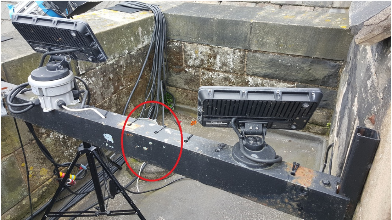
Fig. 4b Edinburgh Castle Gatehouse (South) roof mounting pole clamp point
