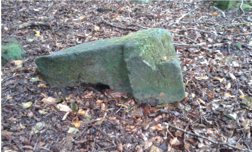
Detached stonework near the well
