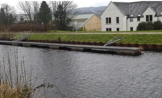
Picture showing one 24m length of refurbished pontoon, to replace the two existing life expired jetty's bellow Lock 4.
