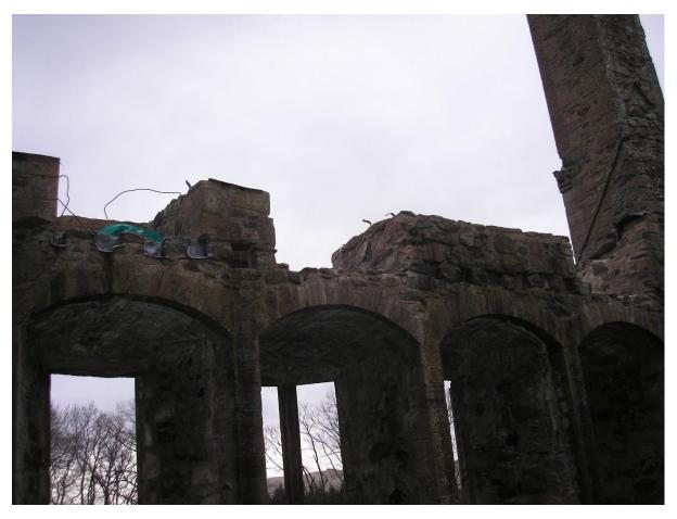
Typical view of section of interior where lead stolen (some pocket flashings remain – to be reinstated).
