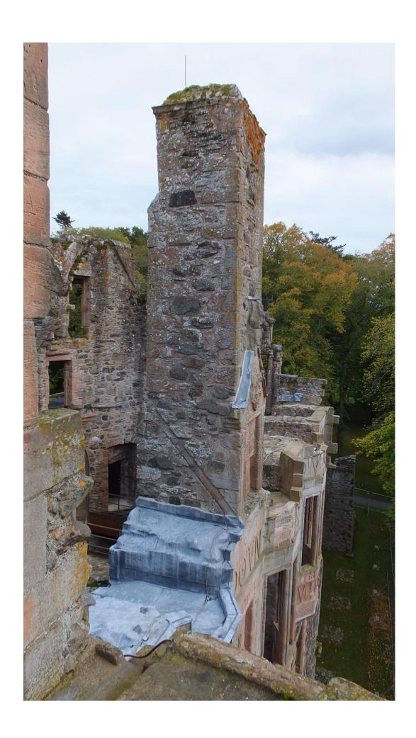
Typical view of wallhead form round tower. Ashlar to front elevation and flashings/drip to interior to be in lead as in previously built scheme (see extract from original drawings).
