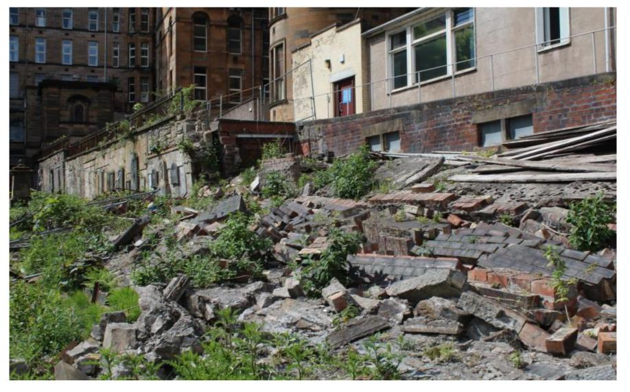
**Being the Restoration of the Fallen Section** - 20 metres of collapsed section of wall and walkway requires completely rebuilt. This damaged section has major Heath and Safety implications
